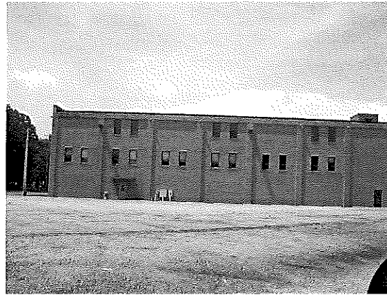
View from the rear of the building.
