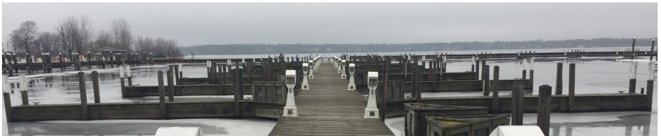
Figure 2: Hartshorn Marina - Center Floating Dock, January, 2017
