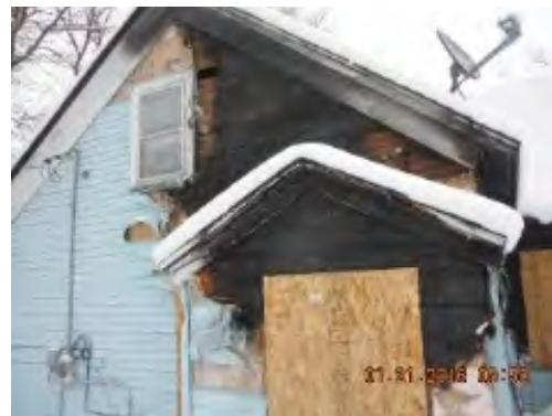
Rear of the structure.
