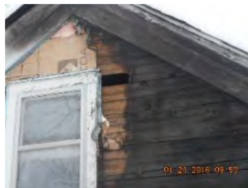
2 nd floor from the rear.
