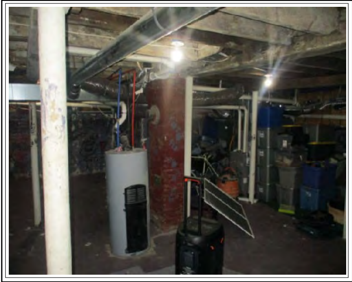
Unfinished Basement (Unit B)
