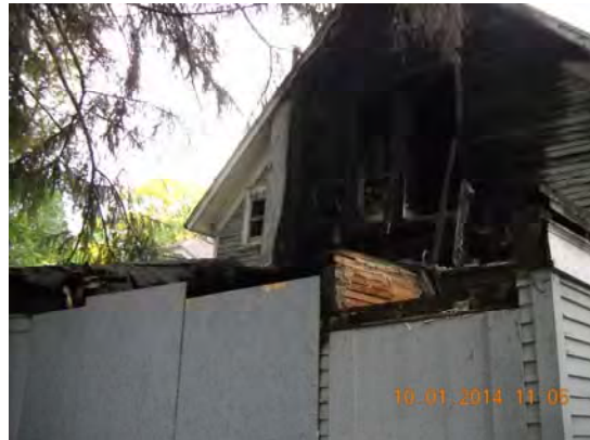
Rear of structure.
