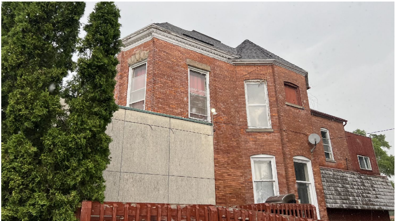
One second-story window (center) on the south elevation proposed to be replaced.
