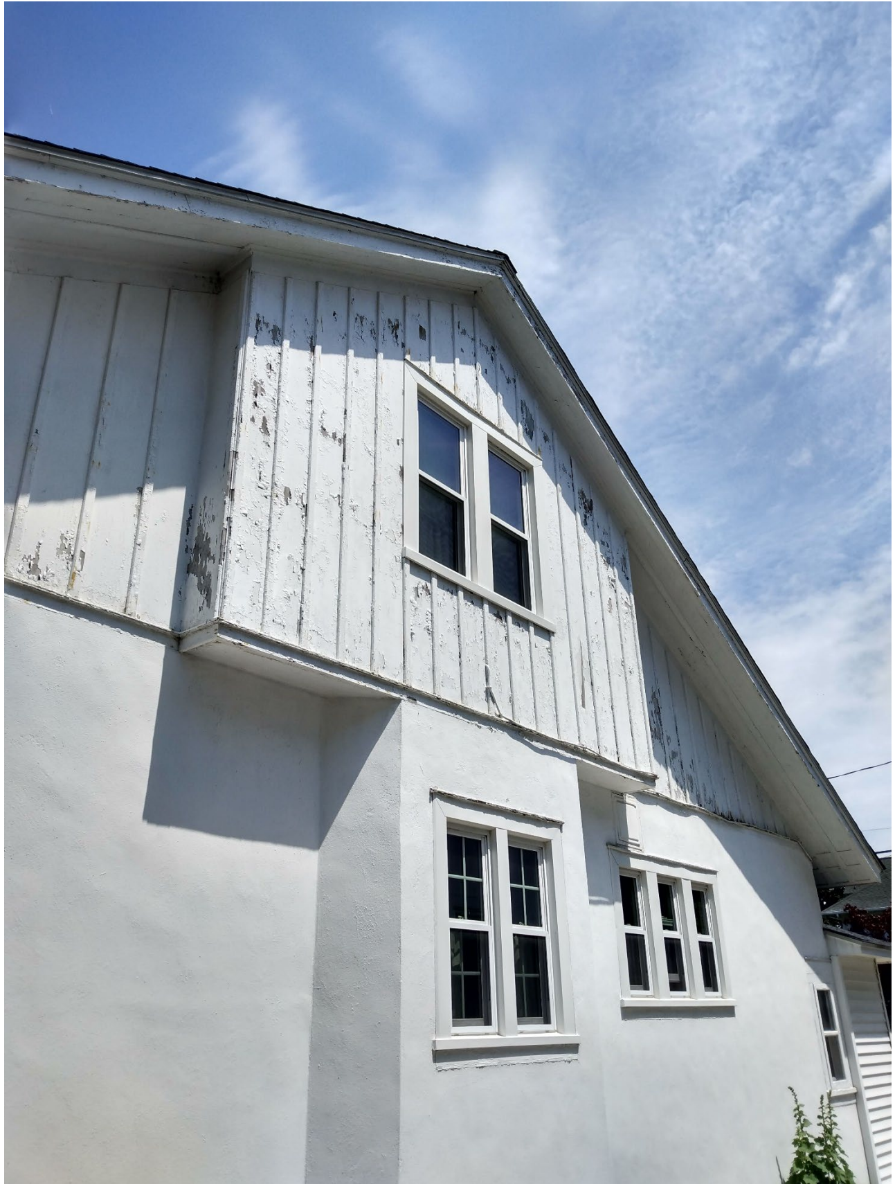
Detail view of the south (side) elevation of the house showing upper portion proposed to be resided.
