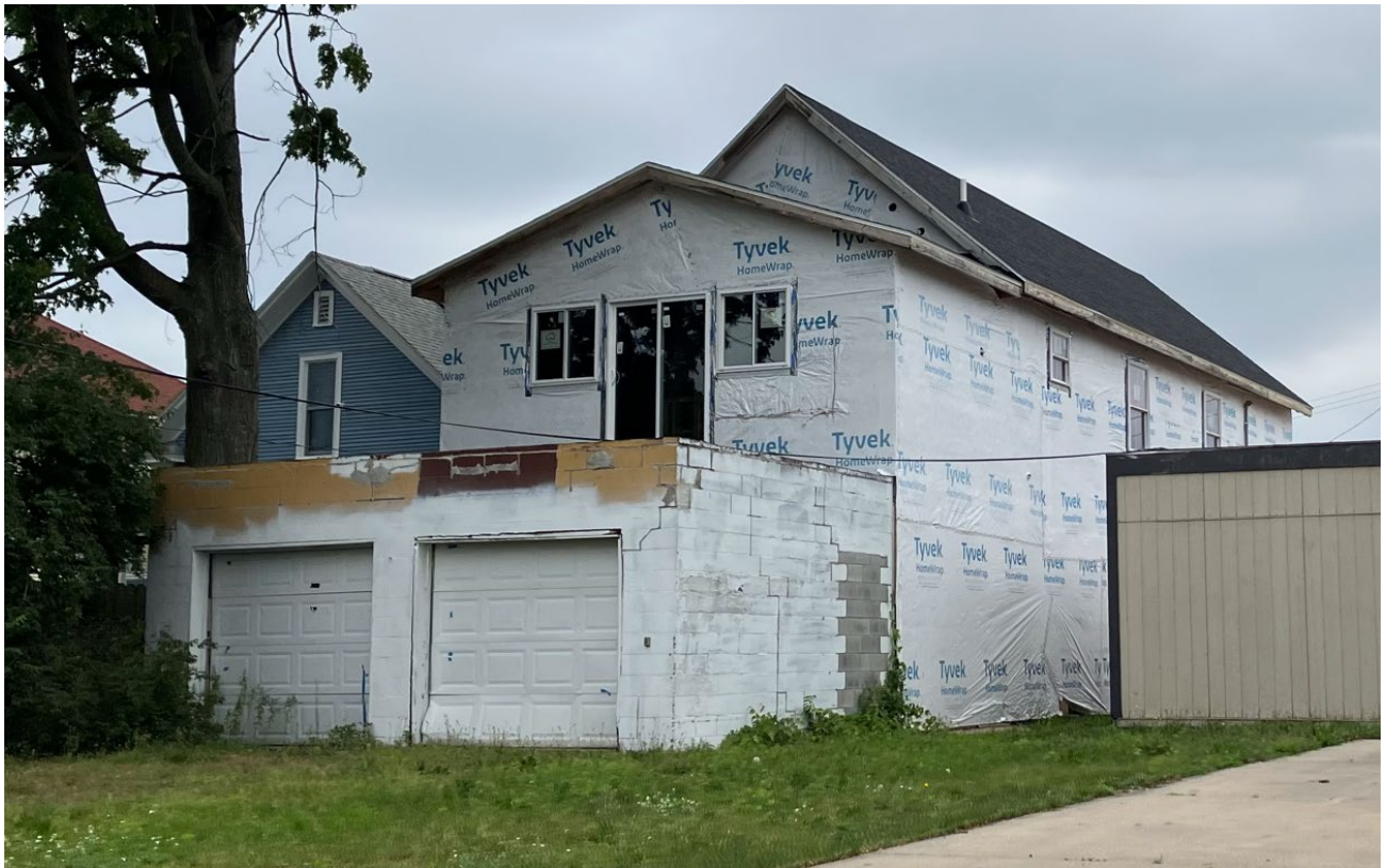
View from rear alley, looking east.
