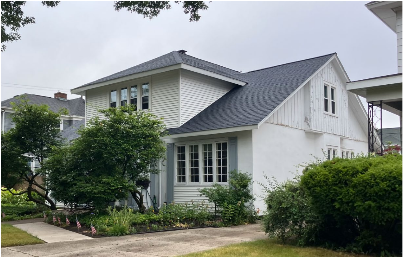
View of the west (front) and south (side) elevations from Peck Street.
