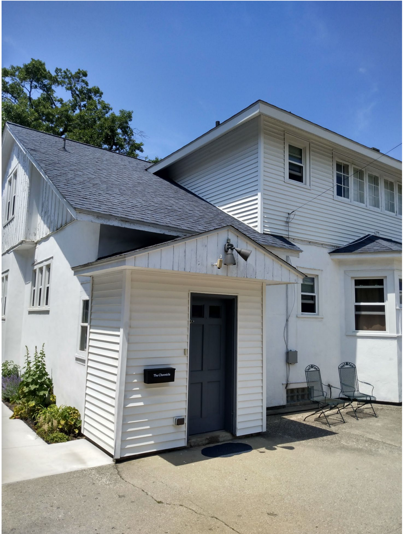
View of the south (side) and east (rear) elevations.
