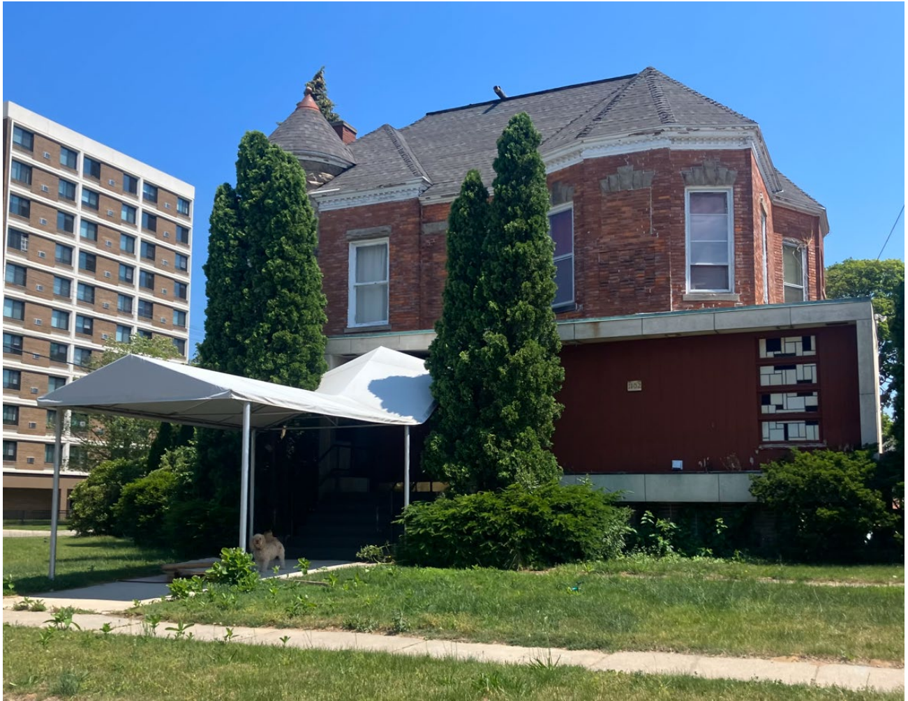
View of house from Terrace Street, looking east.
