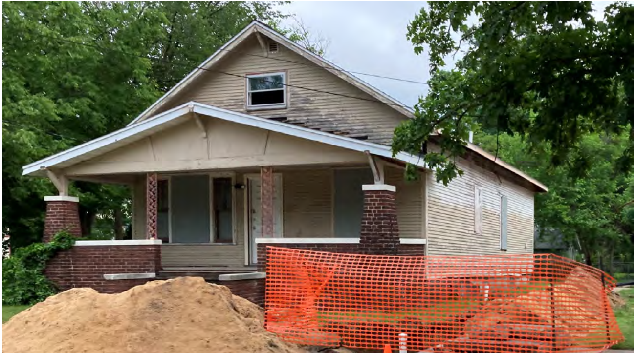
View of south (front) and east (right) elevations from E. Grand Avenue showing window on east elevation to be removed and replaced with a new vinyl egress window in a new location (#2)
