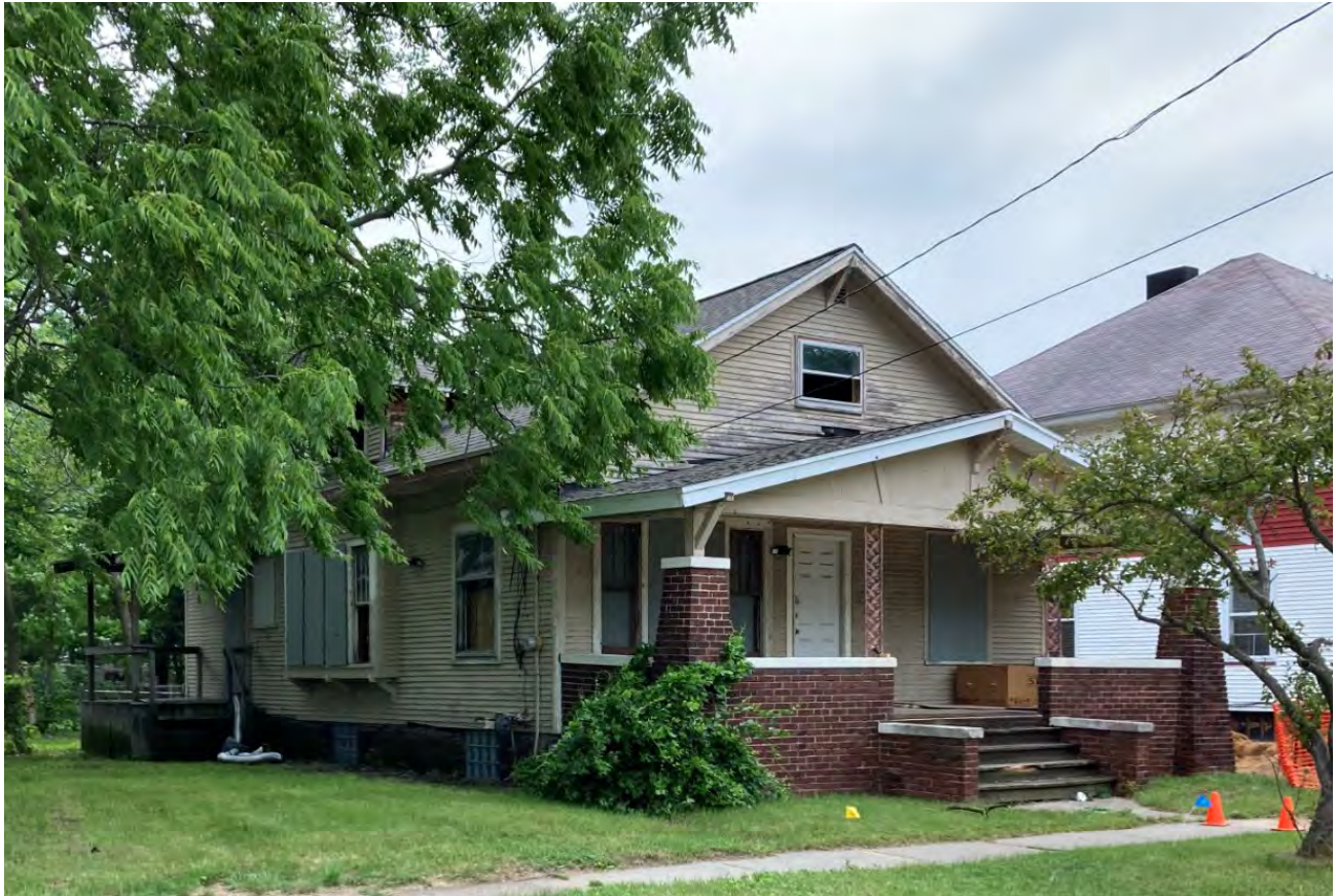
View of south (front) and west (left) elevations from E. Grand Avenue showing second floor window above porch to be replaced with an egress window (#3) and other existing first floor windows to be replaced (#1)
