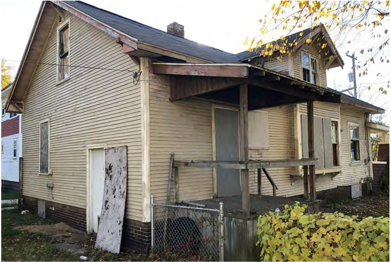
View of north (rear) elevation showing rear door to be eliminated (#5) (photo from fall 2020)
