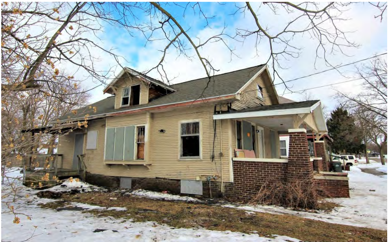
View of west elevation showing location of door to be reversed and replaced (#6) (photo from March 2021)
