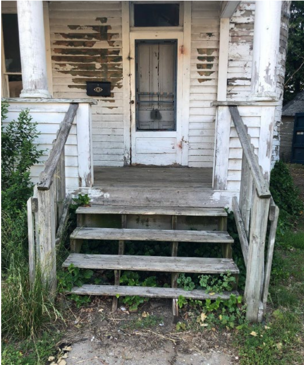
View of existing front steps
