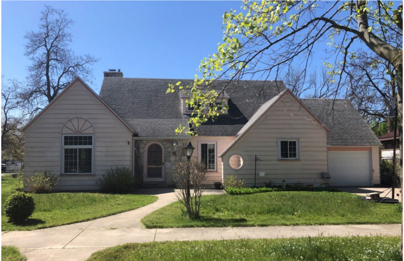
View of house from W. Larch Avenue
