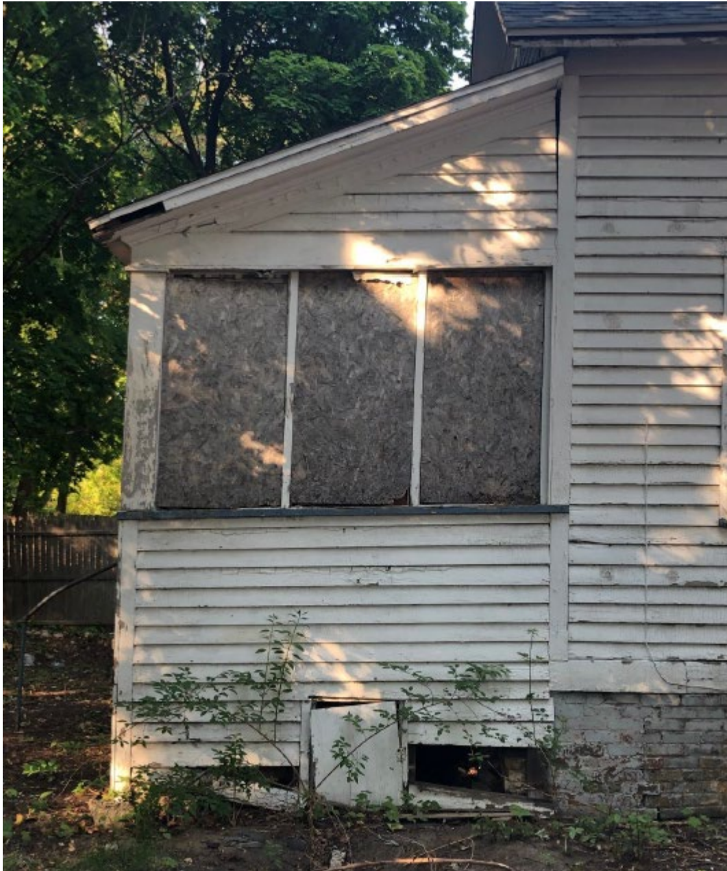
Side view of 8'x18' room to be demolished and rebuilt
