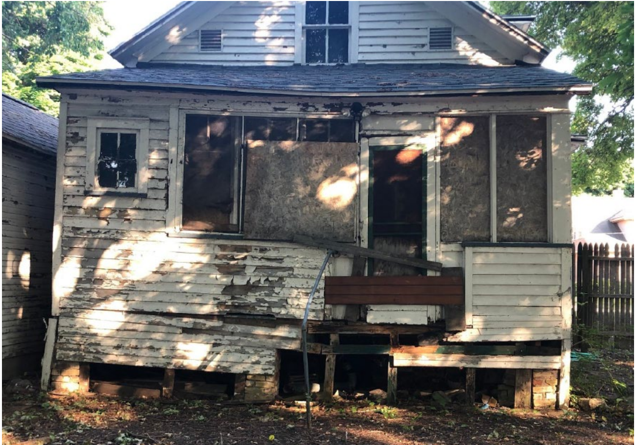
Rear view of 8'x18' room to be demolished and rebuilt
