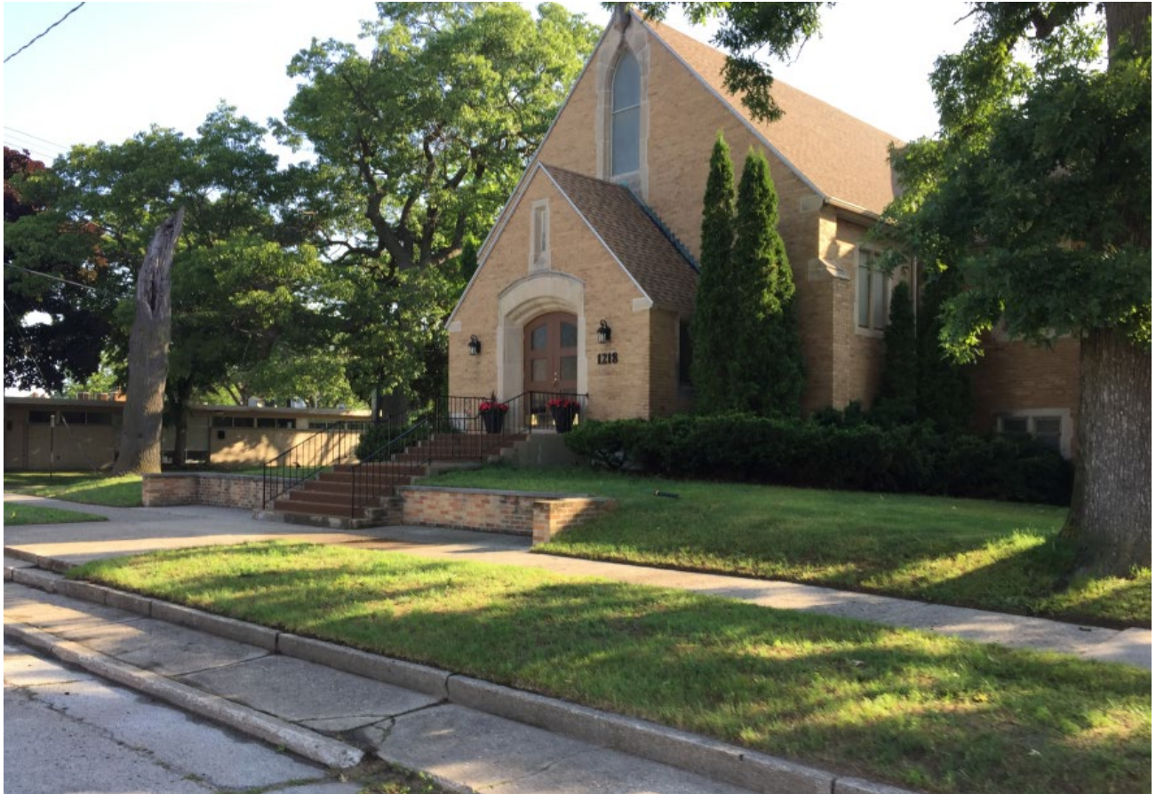
View of structure looking north from Ransom Street
