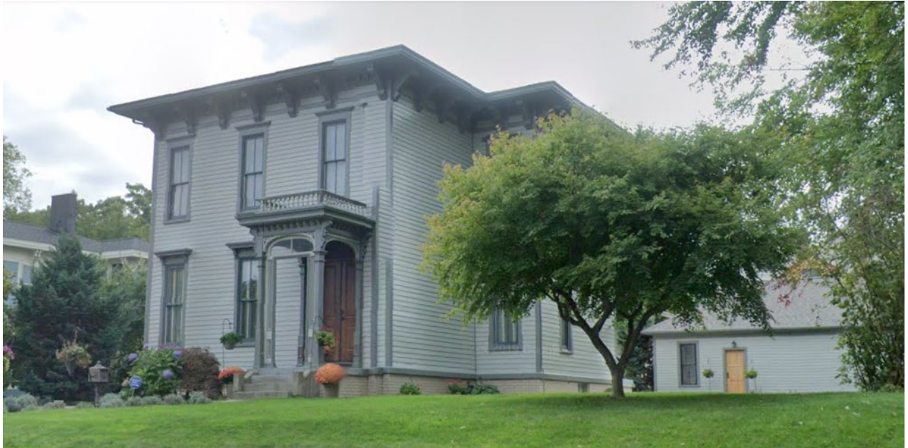
View of house from W. Clay Avenue. Garage door visible at right; side porch not visible from street
