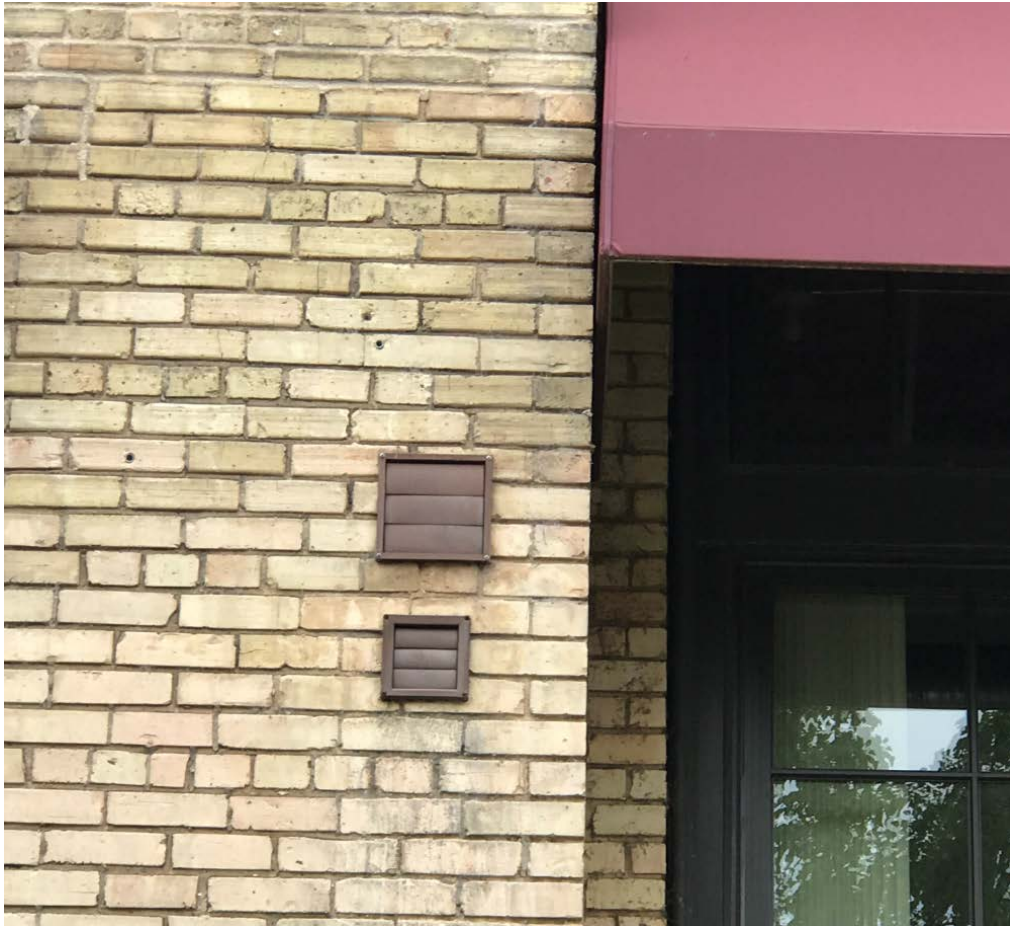
Existing vents on the building
