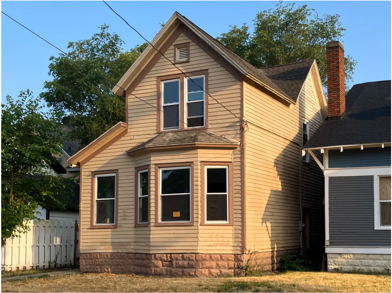
View of house from E. Isabella, looking west.
