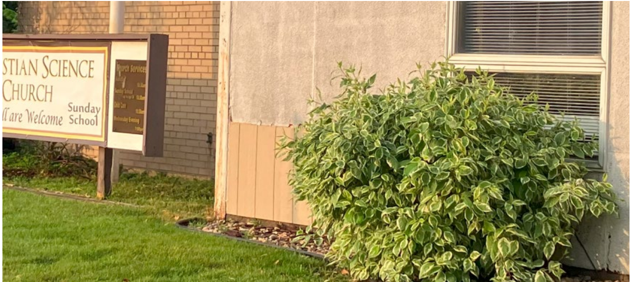
Sample of proposed siding placed on building.
