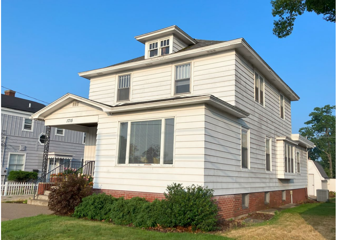
View of the east (front) and north elevations of the house, looking southwest from Peck Street.
