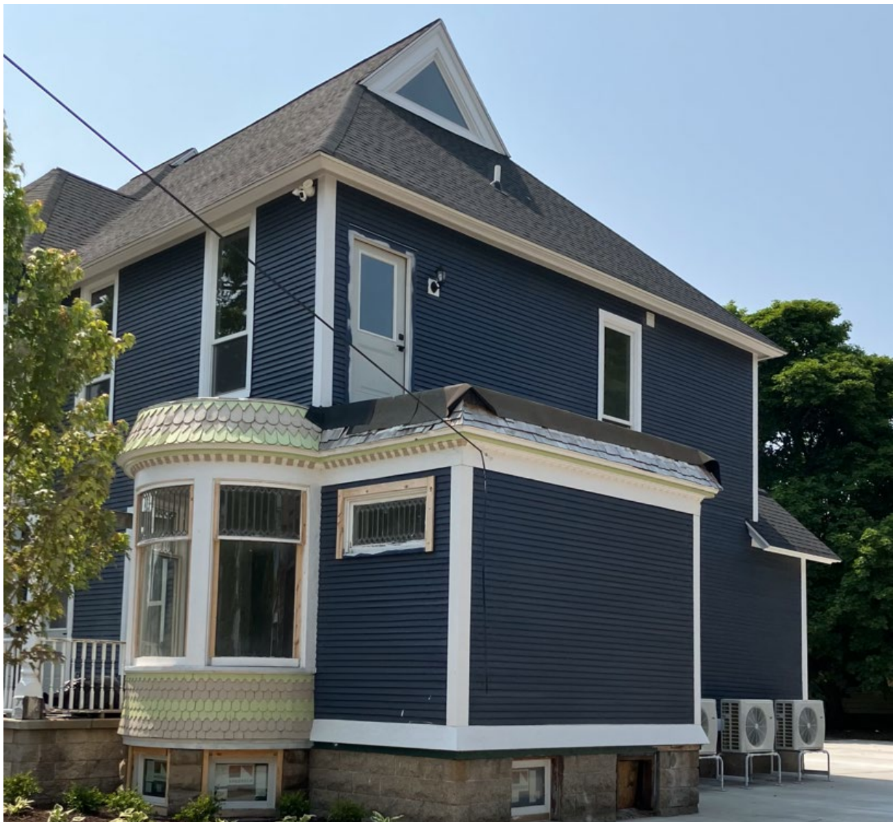
Current view of second story porch on the rear of the house from Delaware Avenue, looking west.
