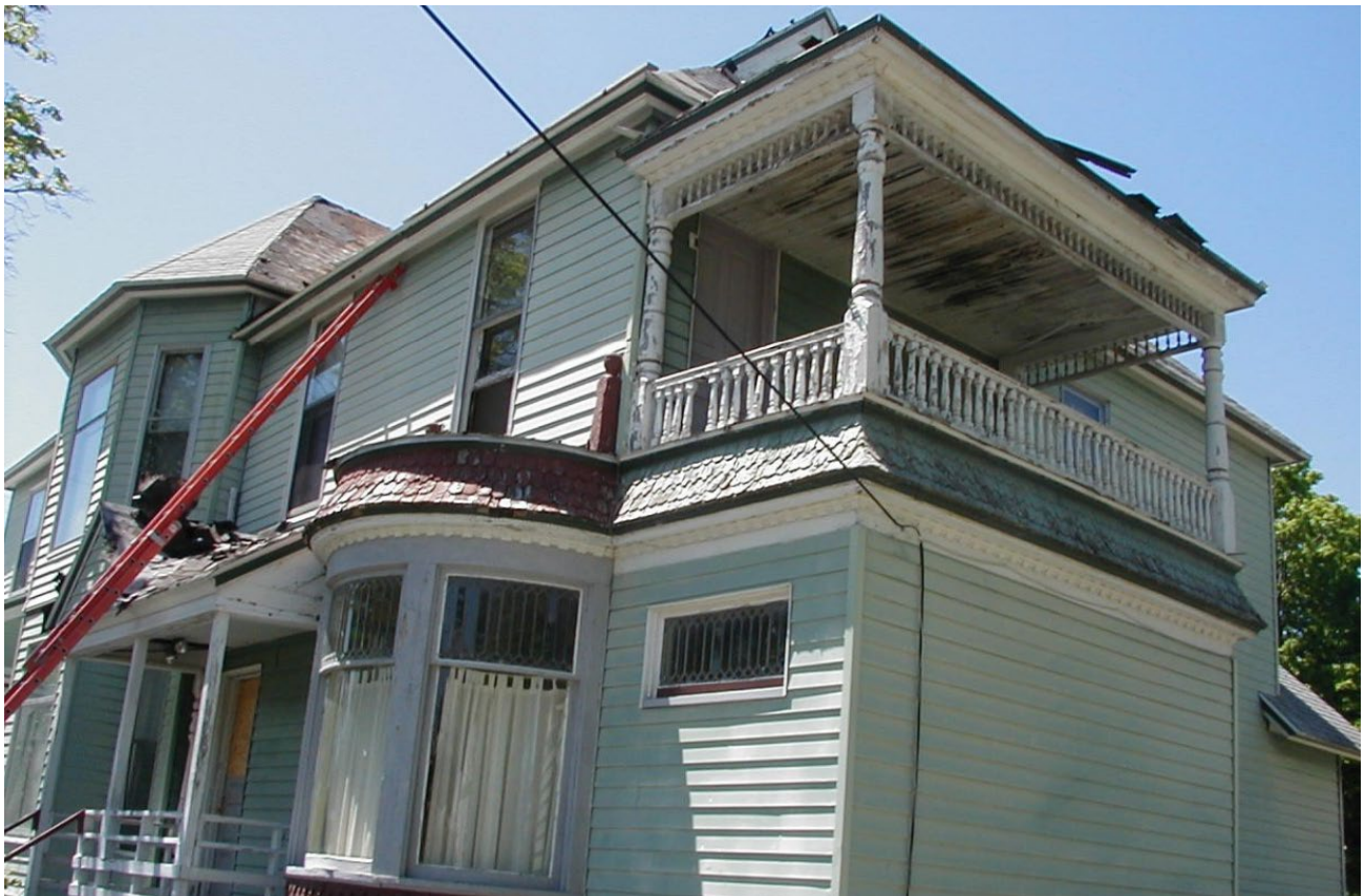
Previous porch railing design including former flat roof (photo from June 2009).
