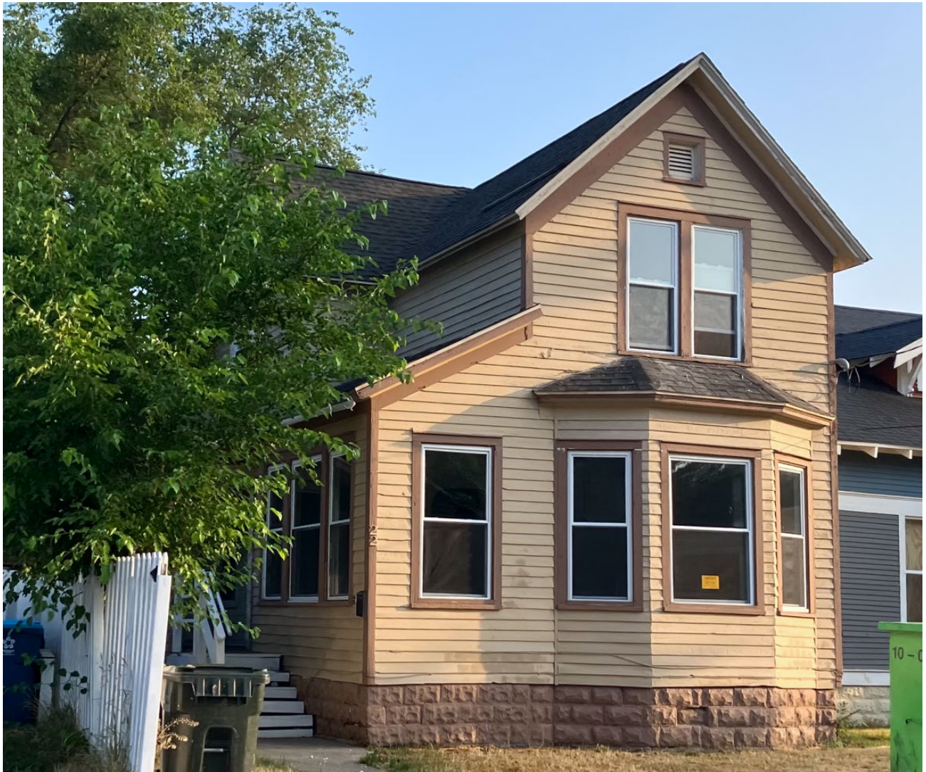
View of house from E. Isabella, looking north.
