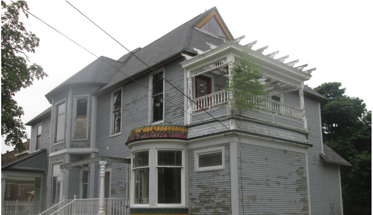
Porch design following the June 2009 HDC approval of a request to “restore and repair the porches in the same style with the railings built to code...and add a gable to the second story porch.” Also reflected in this photo is the October 2009 HDC approval of a pergola-style roof instead of the previously-approved (though never installed) gable roof (photo from July 2021).
