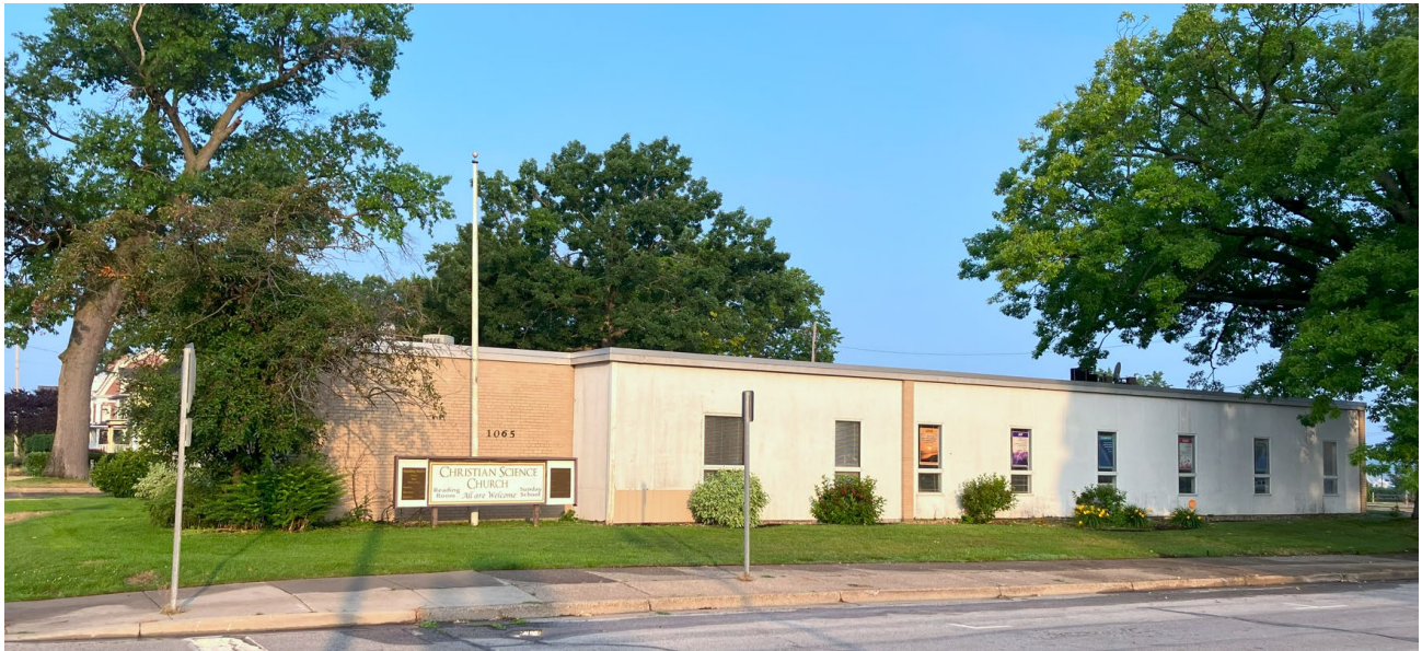
View of building from intersection of W. Webster Avenue and 4 th Street, looking west. All areas with white material are proposed to be replaced.
