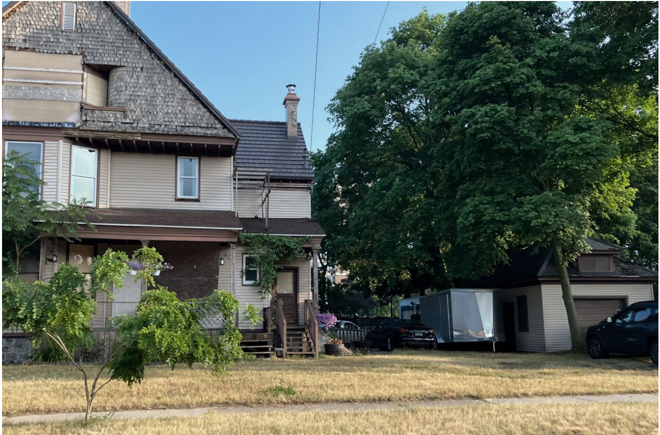
View of existing house and detached garage and proposed location of new garage from Diana Avenue, looking north.
