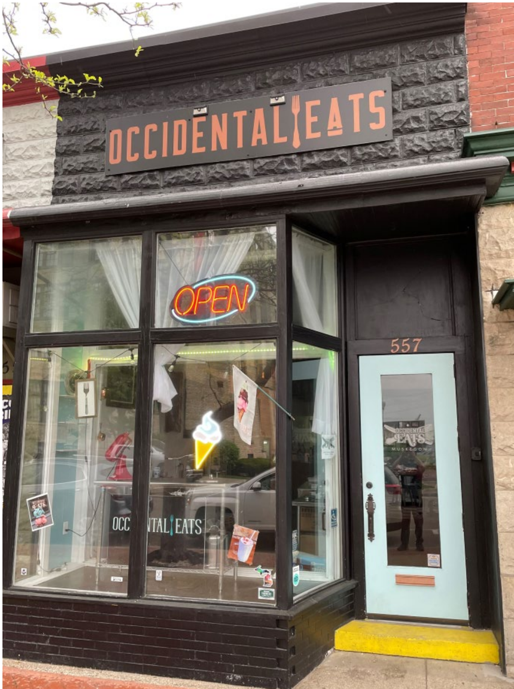
Existing conditions on the W. Western Avenue elevation.
