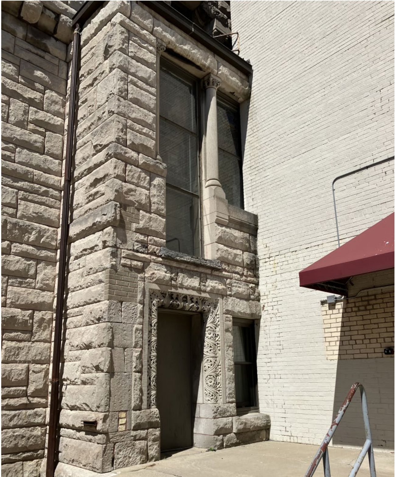
Closer view of connection point between original house and building addition from rear entry to building addition.
