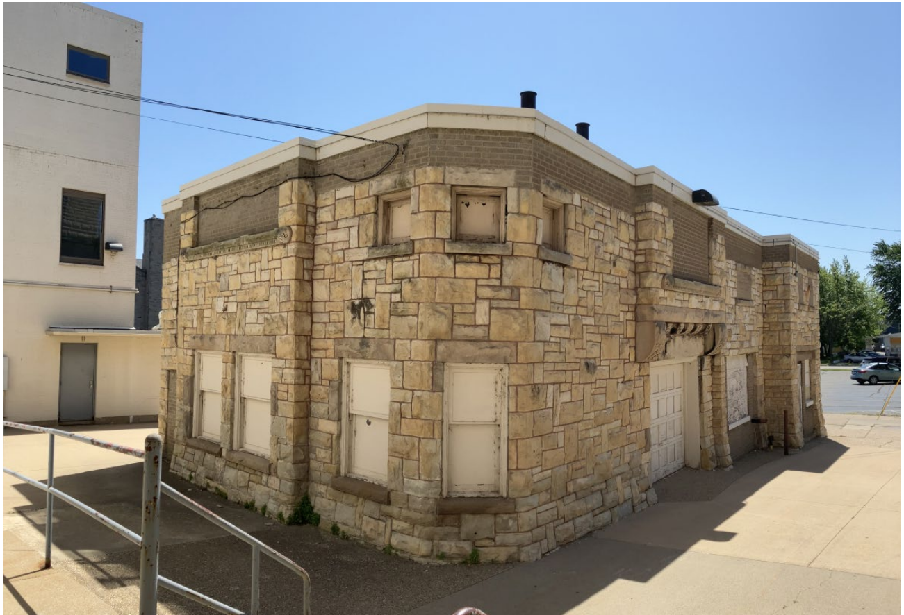
View of carriage house from rear entry to building addition, looking east.
