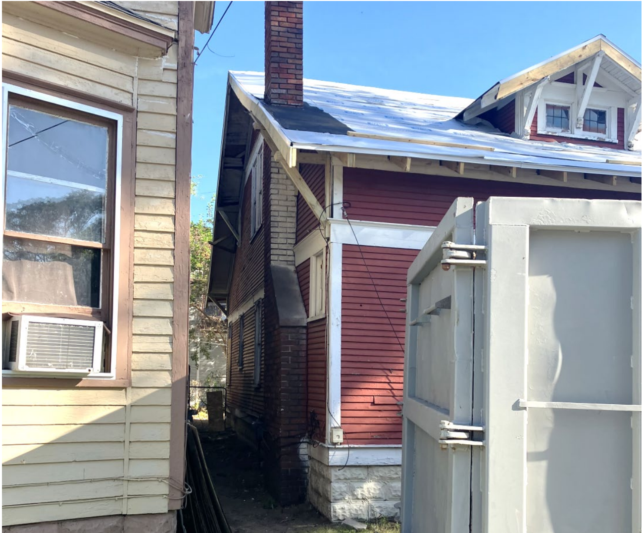
View of windows on side of house and dormer windows, looking north.
