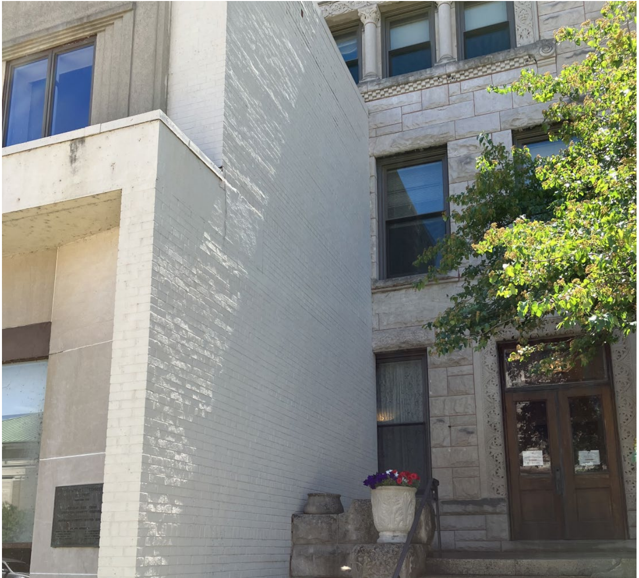
View of connection point between original house and building addition from W. Webster Avenue.
