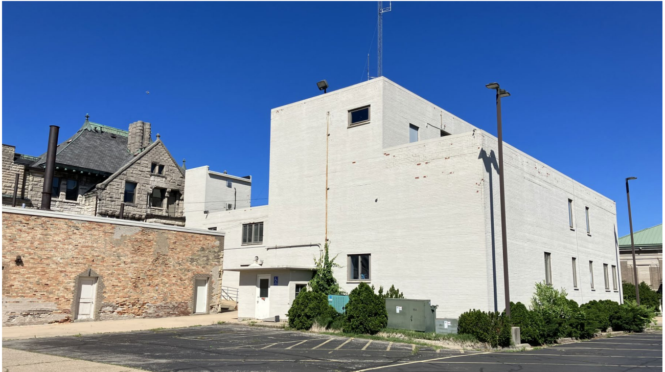
View of carriage house (left) and building addition (right), looking west.
