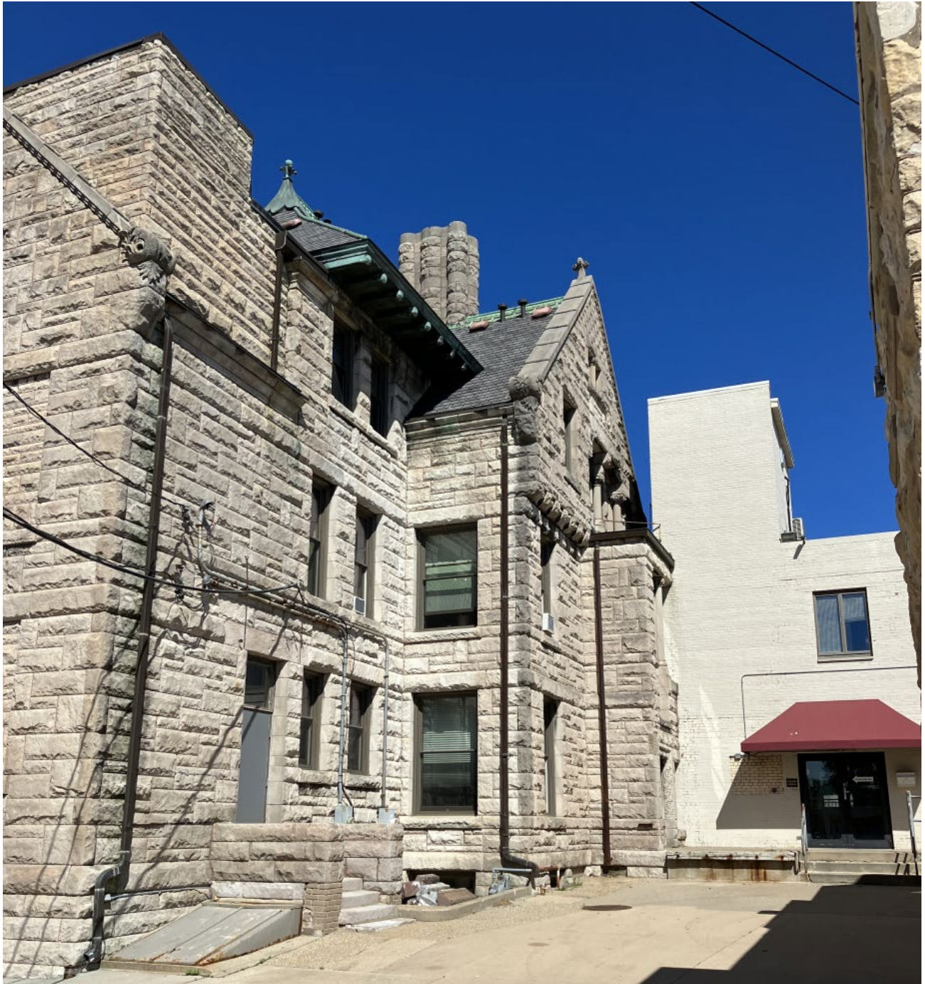
View of rear entry to building addition and connection point to original house, looking west.
