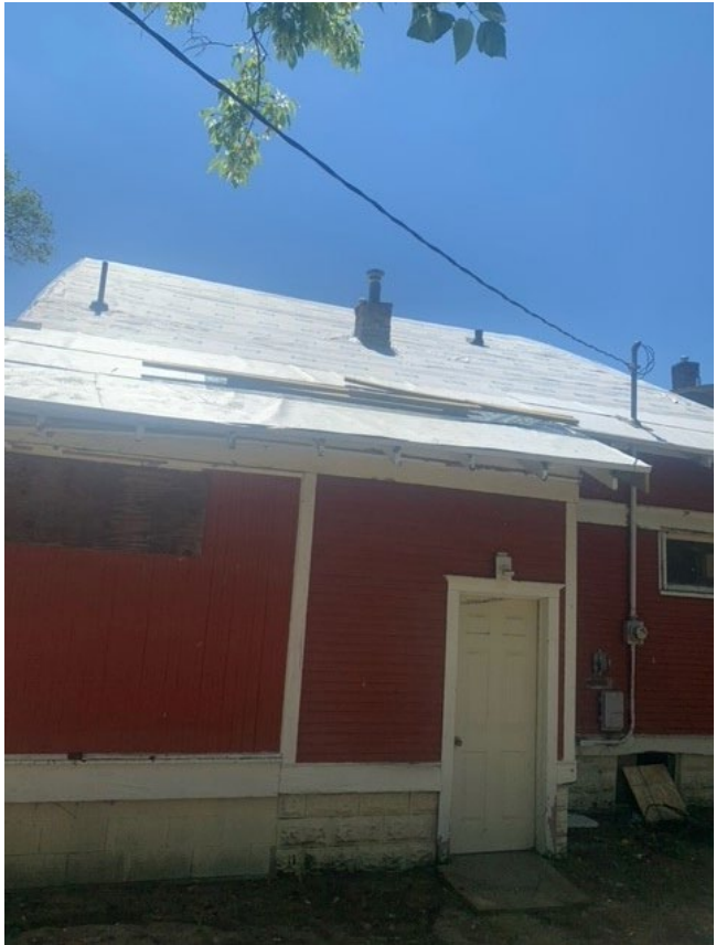
View of the rear elevation of the house from the back yard. Missing window proposed to be removed visible at left and existing basement window proposed to be replaced with a larger window and window-well for egress at right. Upper right window proposed to be replaced with vinyl window of the same size.
