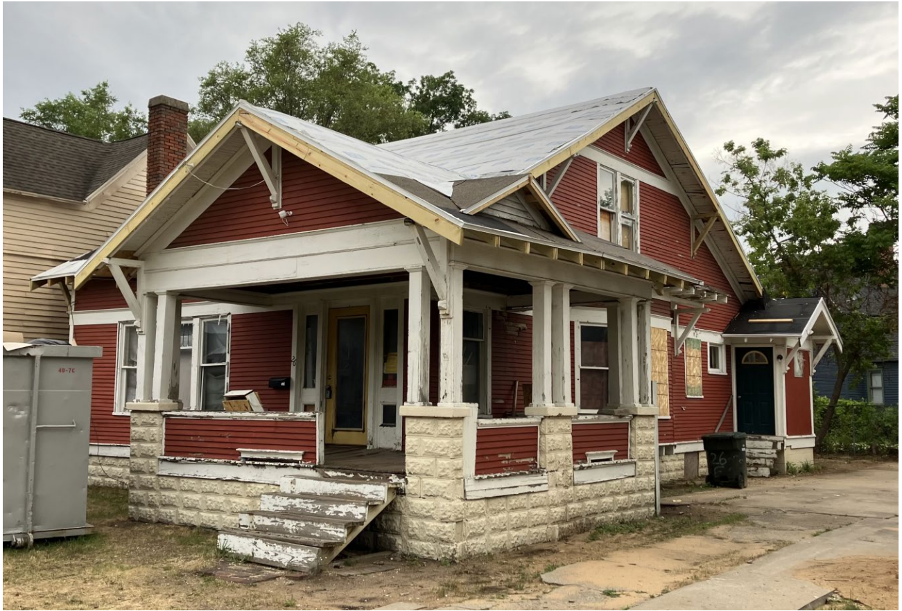
View of house showing windows on side elevation, looking west.
