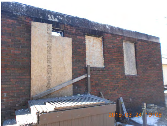
Rear of the structure.
