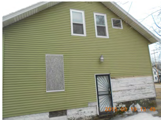
Rear of structure.
