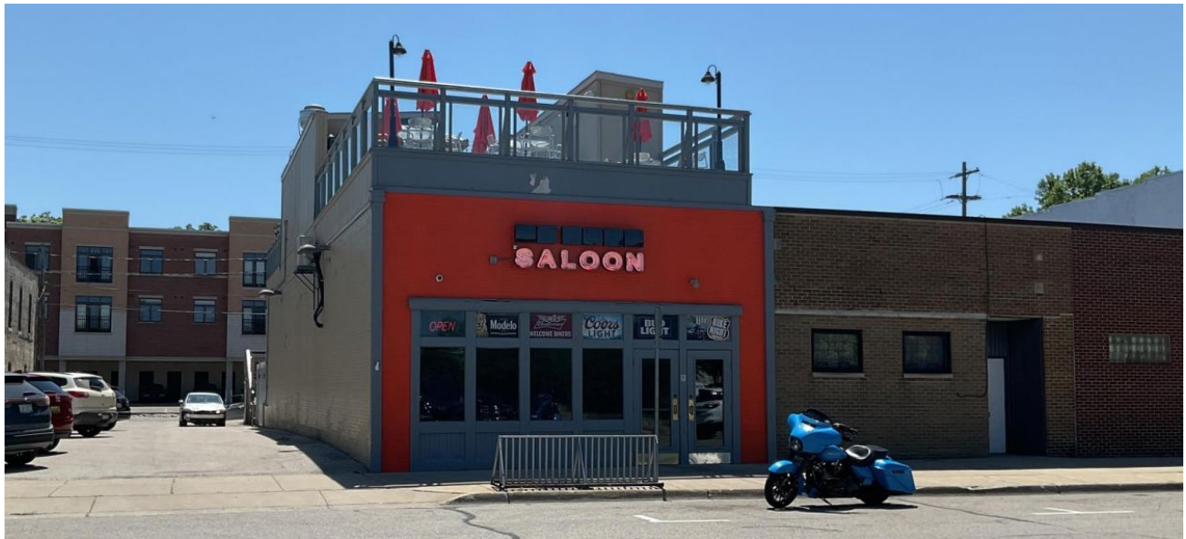
View of the north (front) elevation prior to completion of work, looking south from W. Western Avenue (photo from June 2022).
