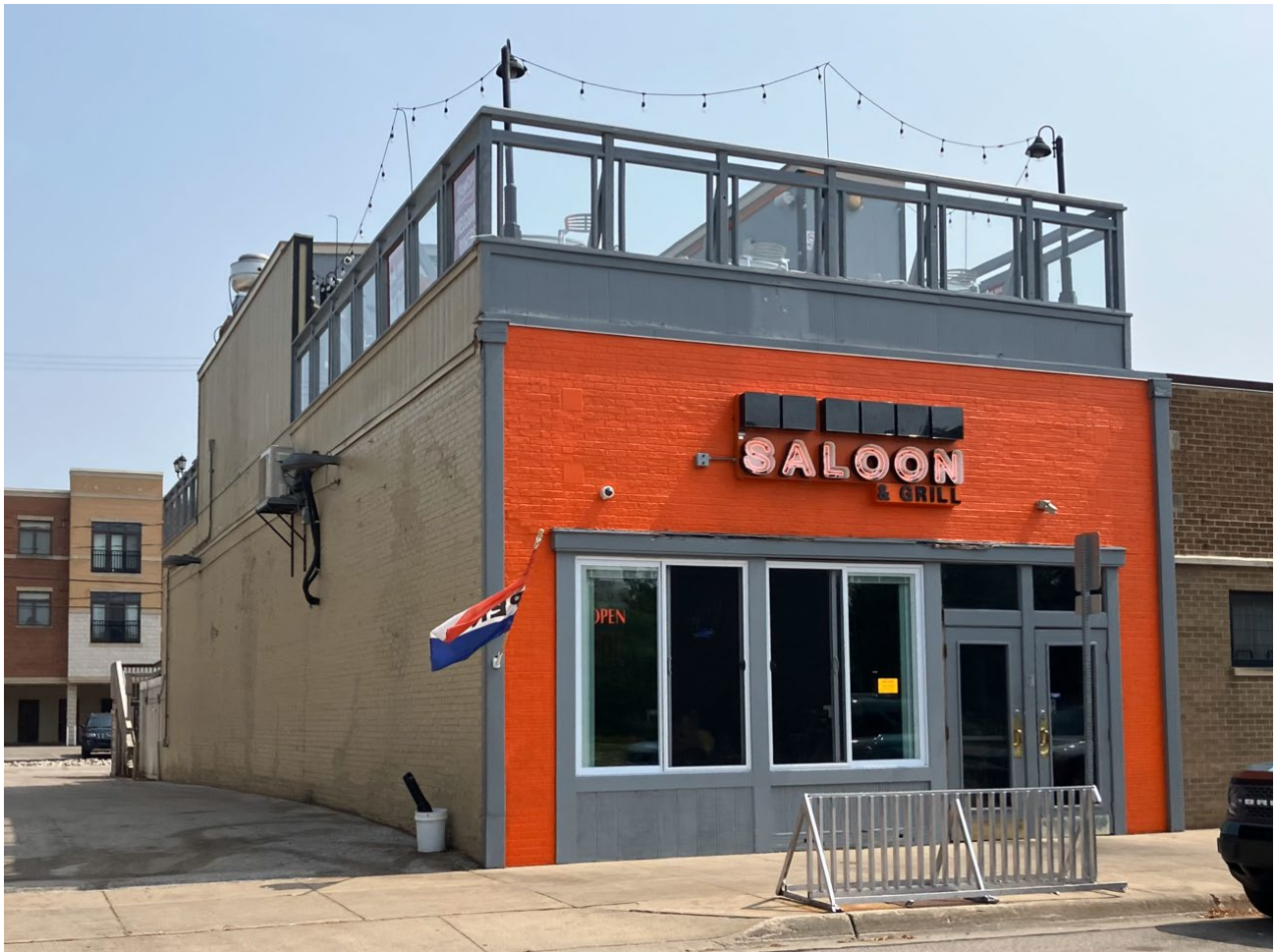
Current view of north elevation.
