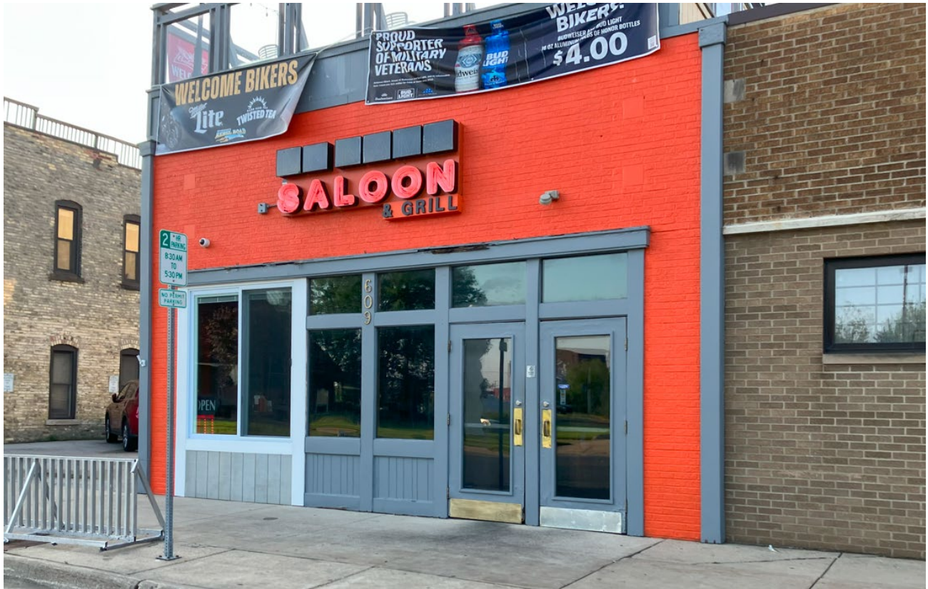
View of north elevation showing partially completed work.
