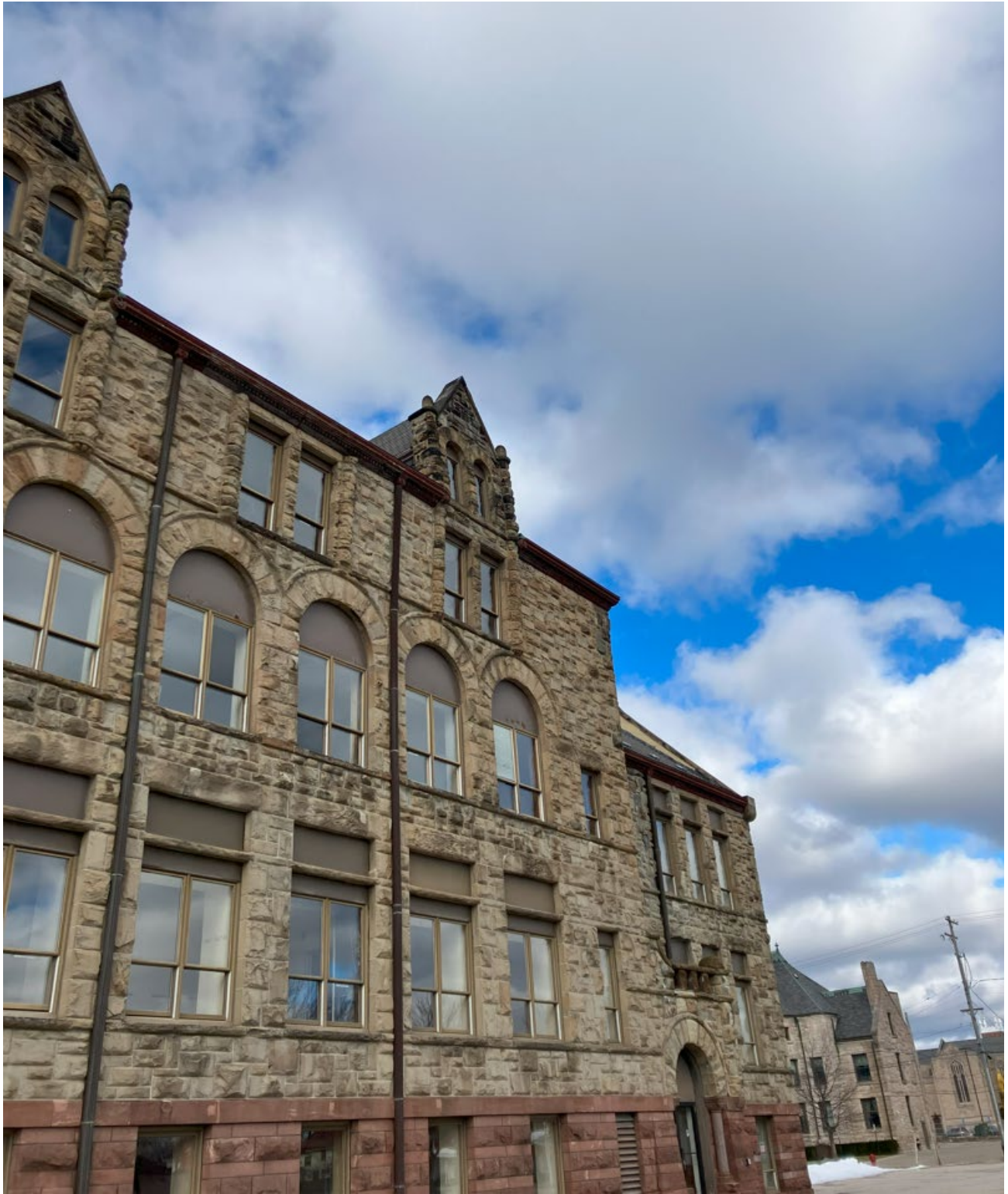
View of south wall from parking lot (photo from February 2023).
