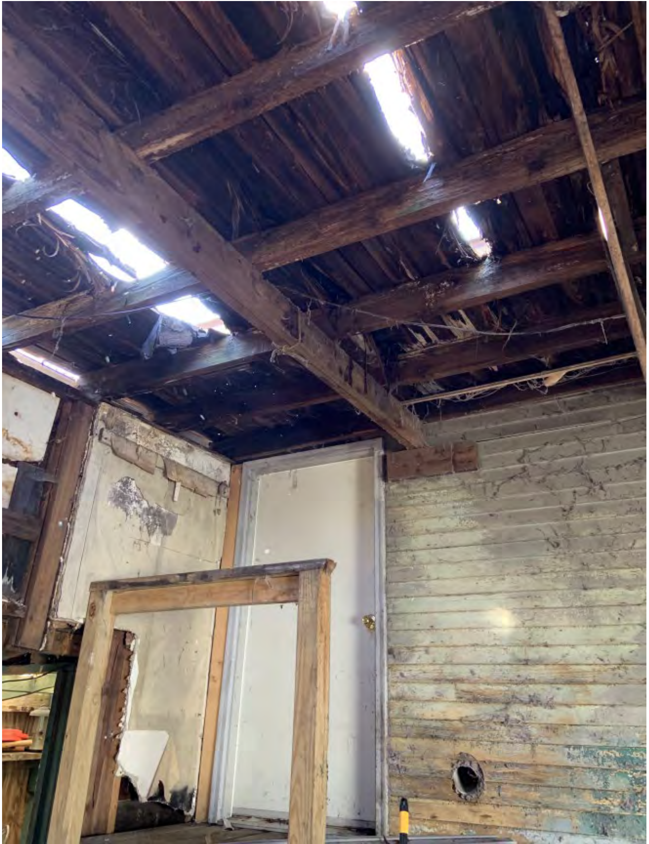
Interior condition of garage and connection to house
