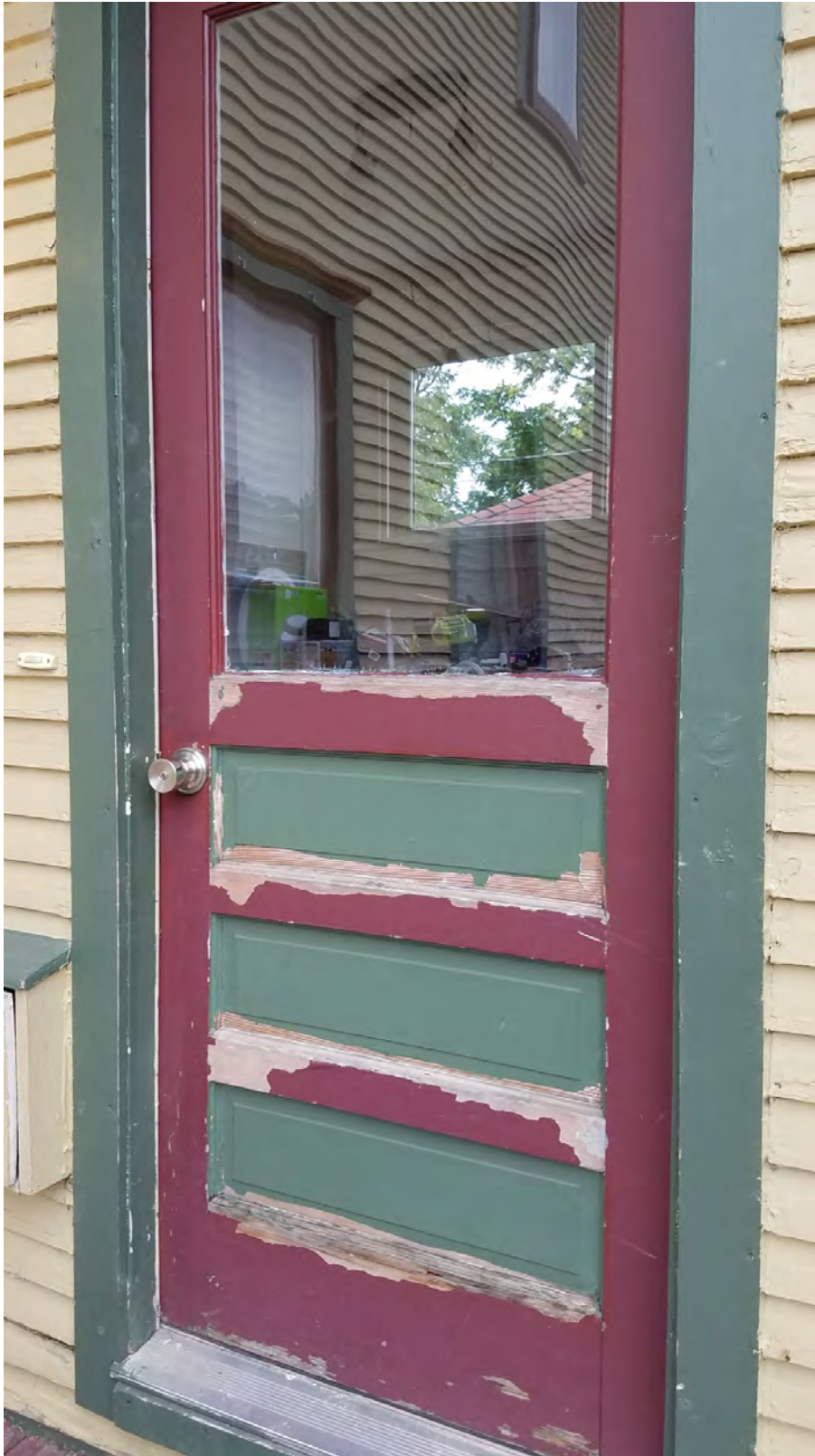
Rear side entry door
