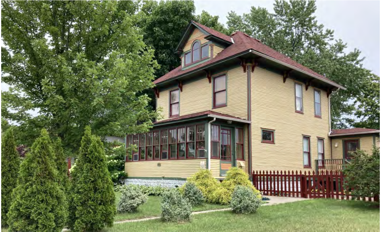
View of house from W. Webster Avenue, rear side entry door visible at right
