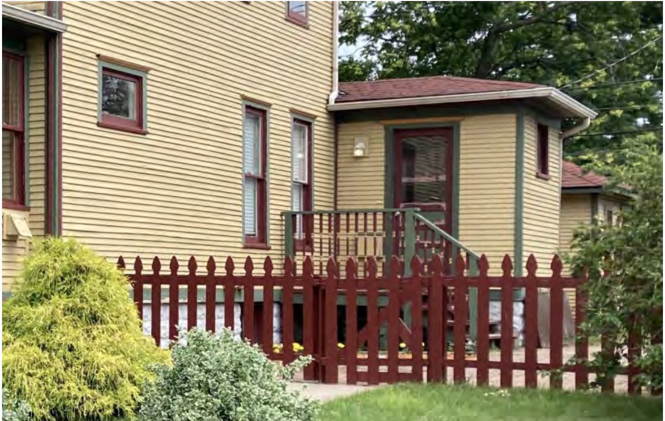
View of rear side entry door and garage from W. Webster
