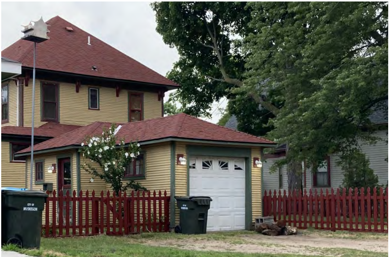
View of garage from alley, garage entry door to be replaced is visible at left
