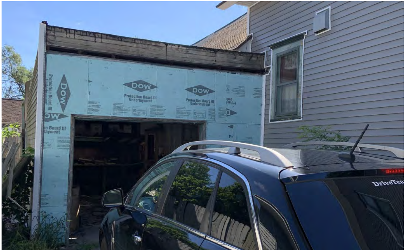
View of garage from driveway and vinyl siding to be matched if garage is demolished
