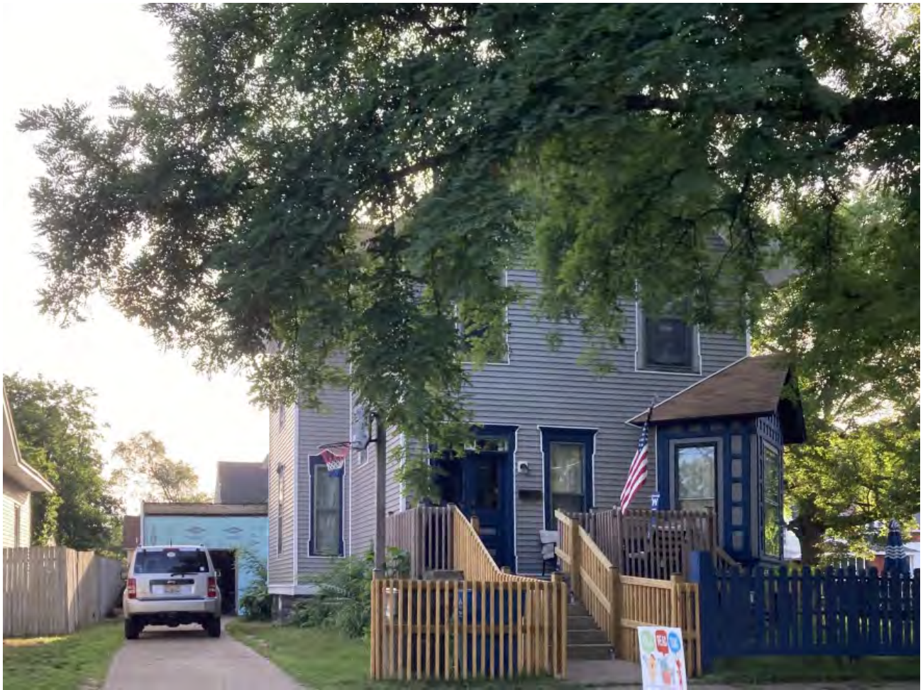
View of structure from Ransom Street, garage visible at left.
