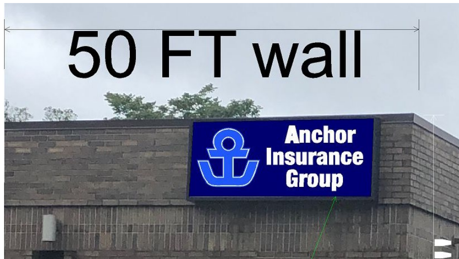
Sign face to be installed in existing sign frame on south façade
