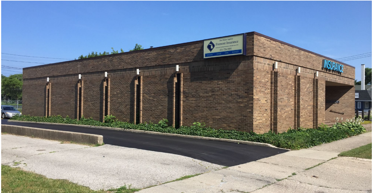
View from Peck showing both signs to be replaced
