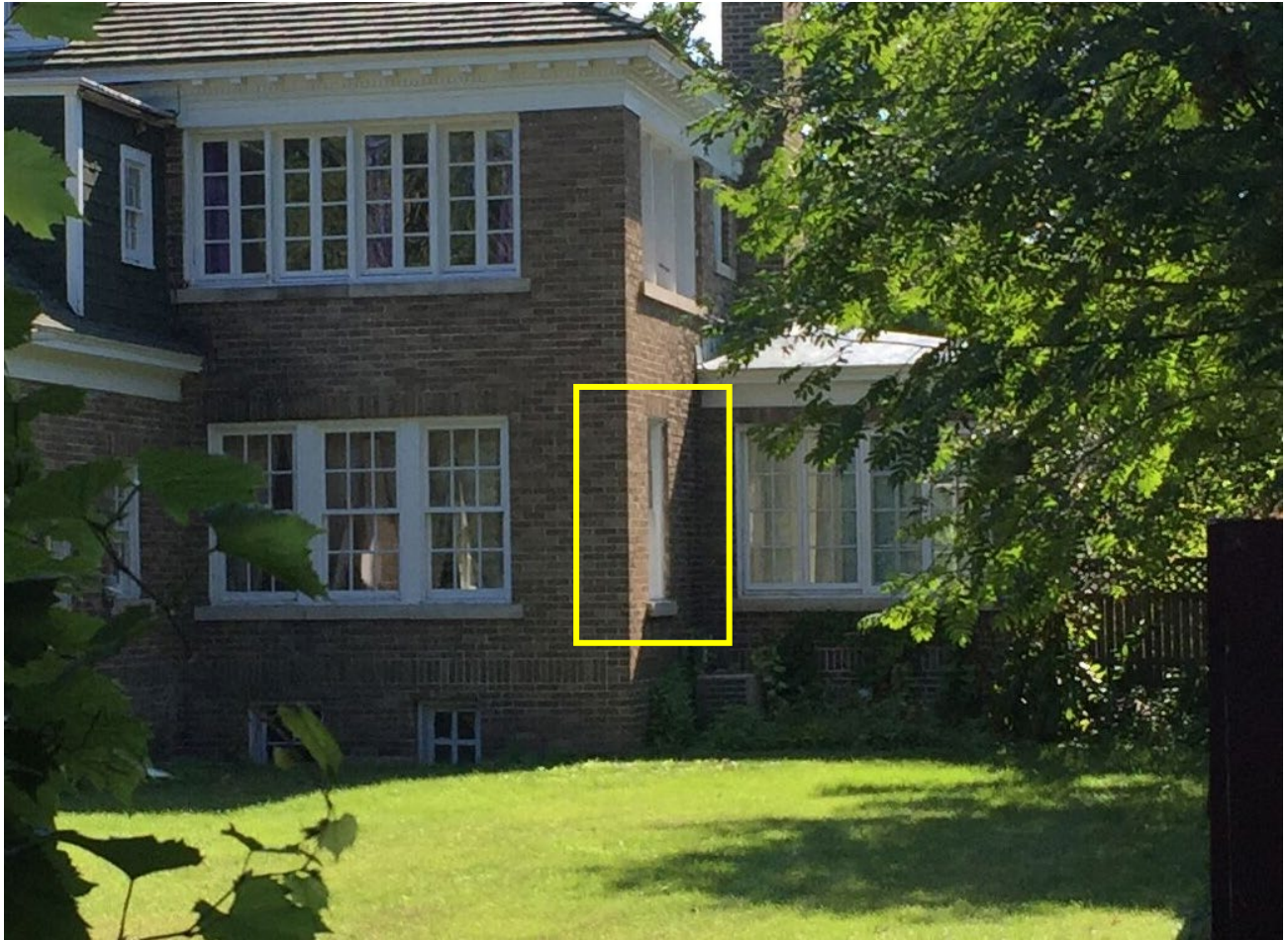
South-facing window to be replaced with door (viewed from alley)
