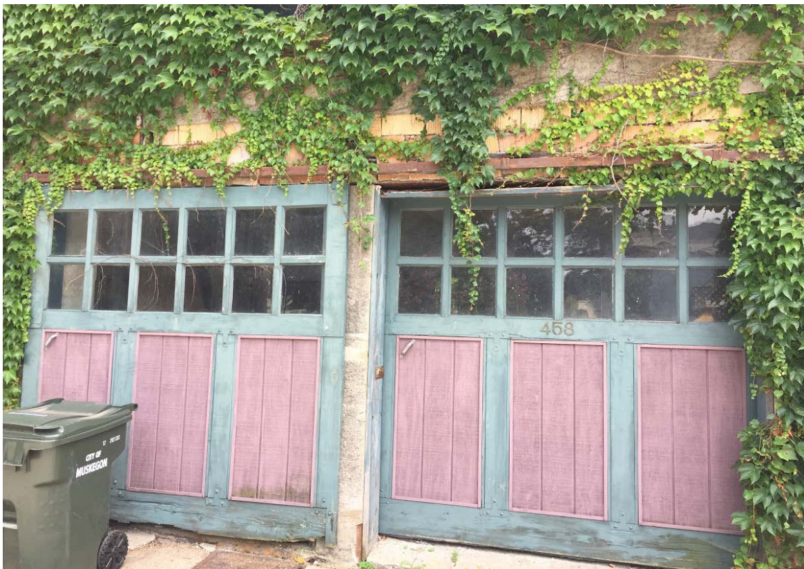
Current condition of rear wall, exposed clay masonry blocks where former awning attached
