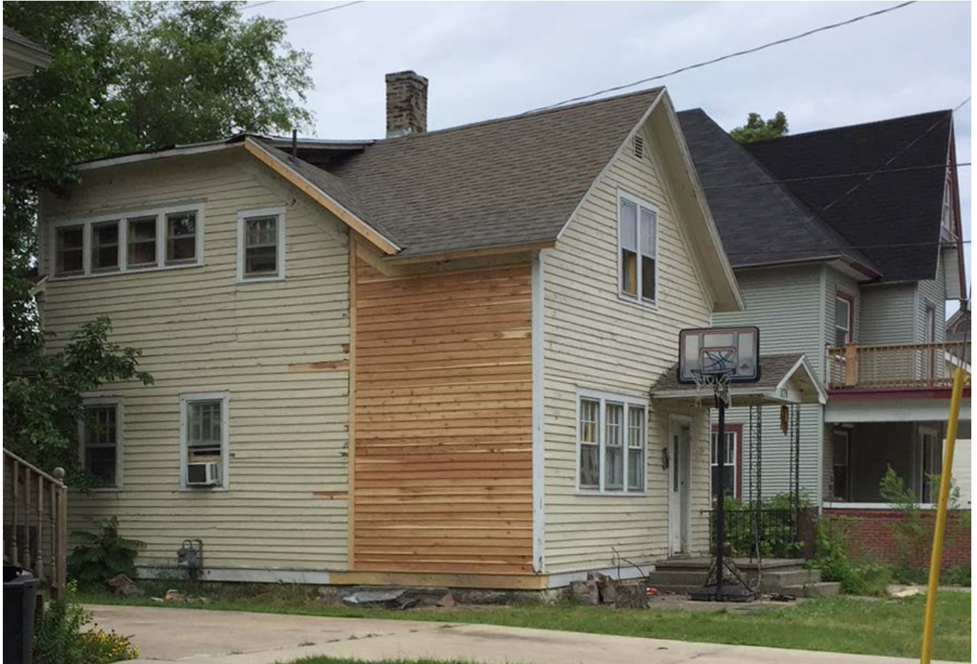
House during chimney repairs
