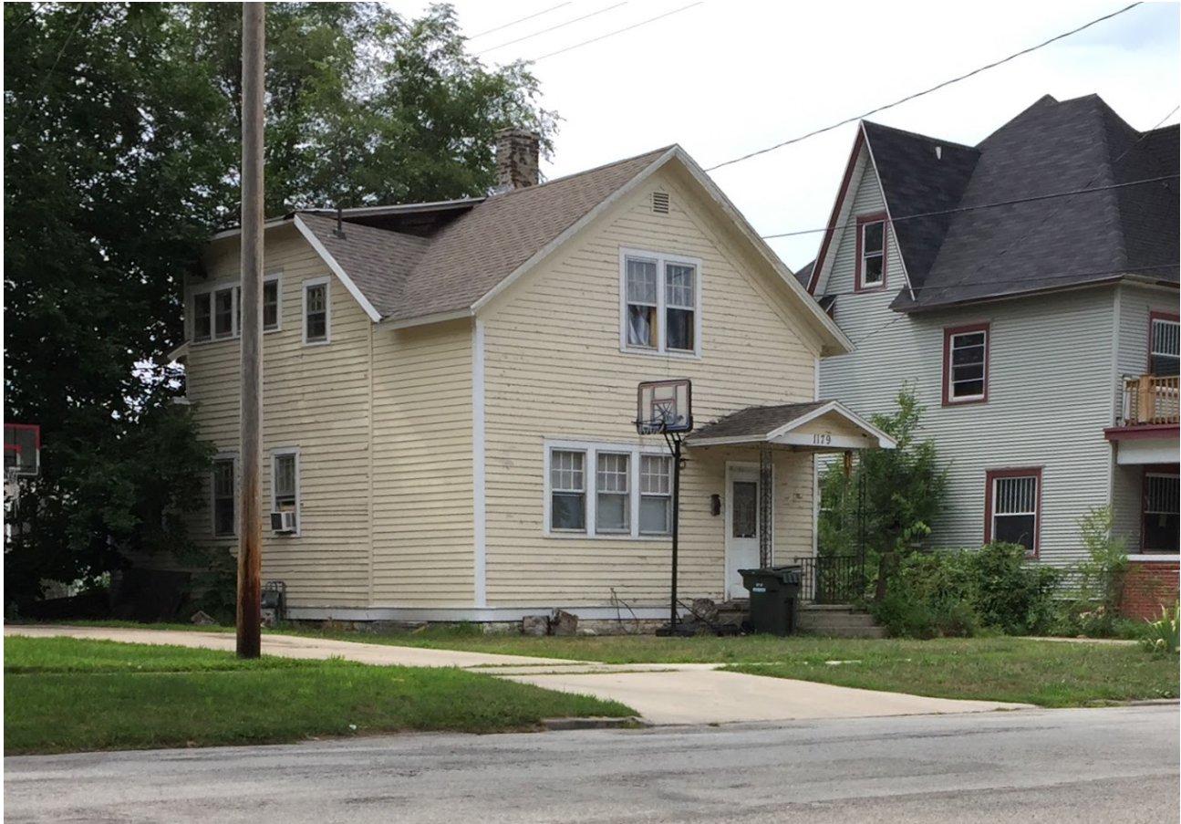
House after chimney removal and repairs to siding
