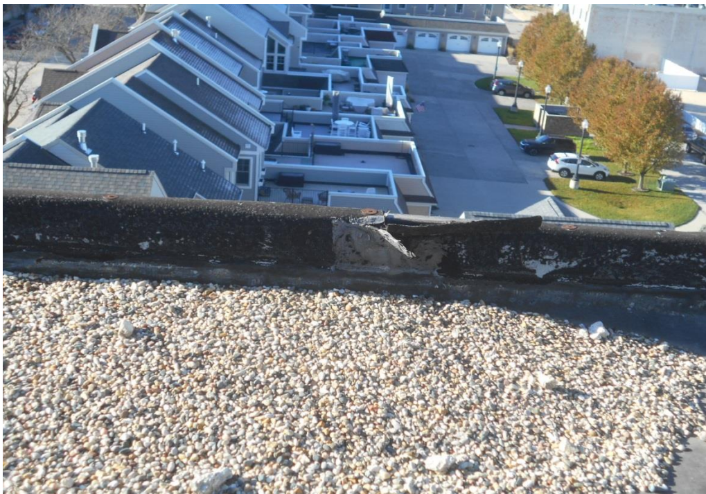
HA #7. Tar and Flashing around Perimeter of Older Building Roof.
