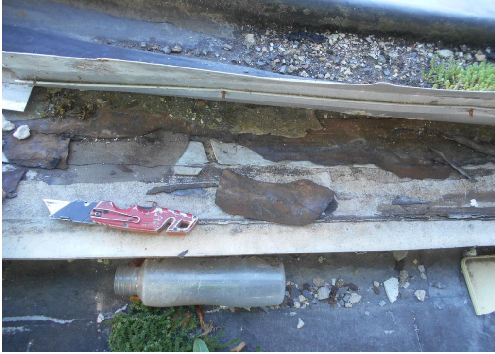
HA #23. Building Sealant (Gray) and Tar Layer (Black). 2 nd Floor/Newer Addition Roof, below rubber roofing membrane.
