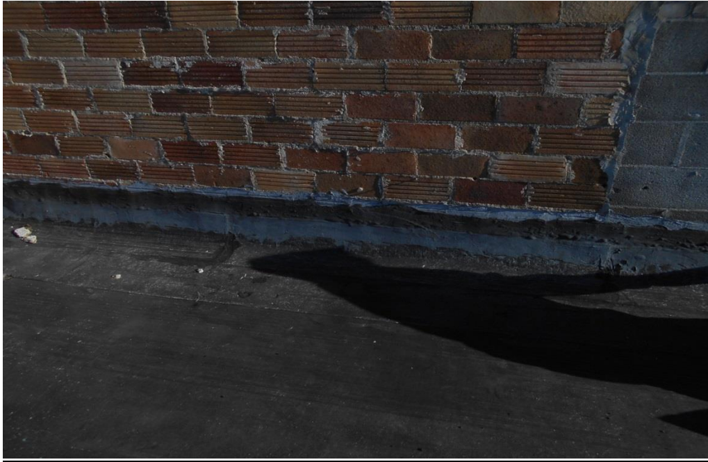
HA #1. Tar and Flashing Layers. On and Around Rooftop Elevator/Mechanical Room.
