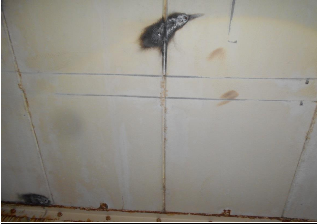
HA #47. Building Caulk, White. Between Precast Concrete Roof and Ceiling Decking on Newer Section of the Building.
