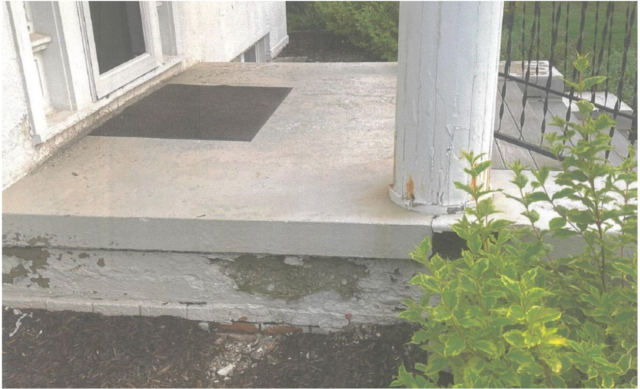
Detail view left side of front porch.
