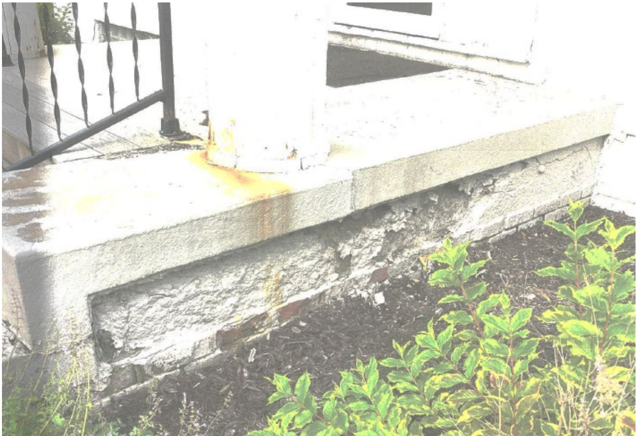
Detail view of right side of front porch.
