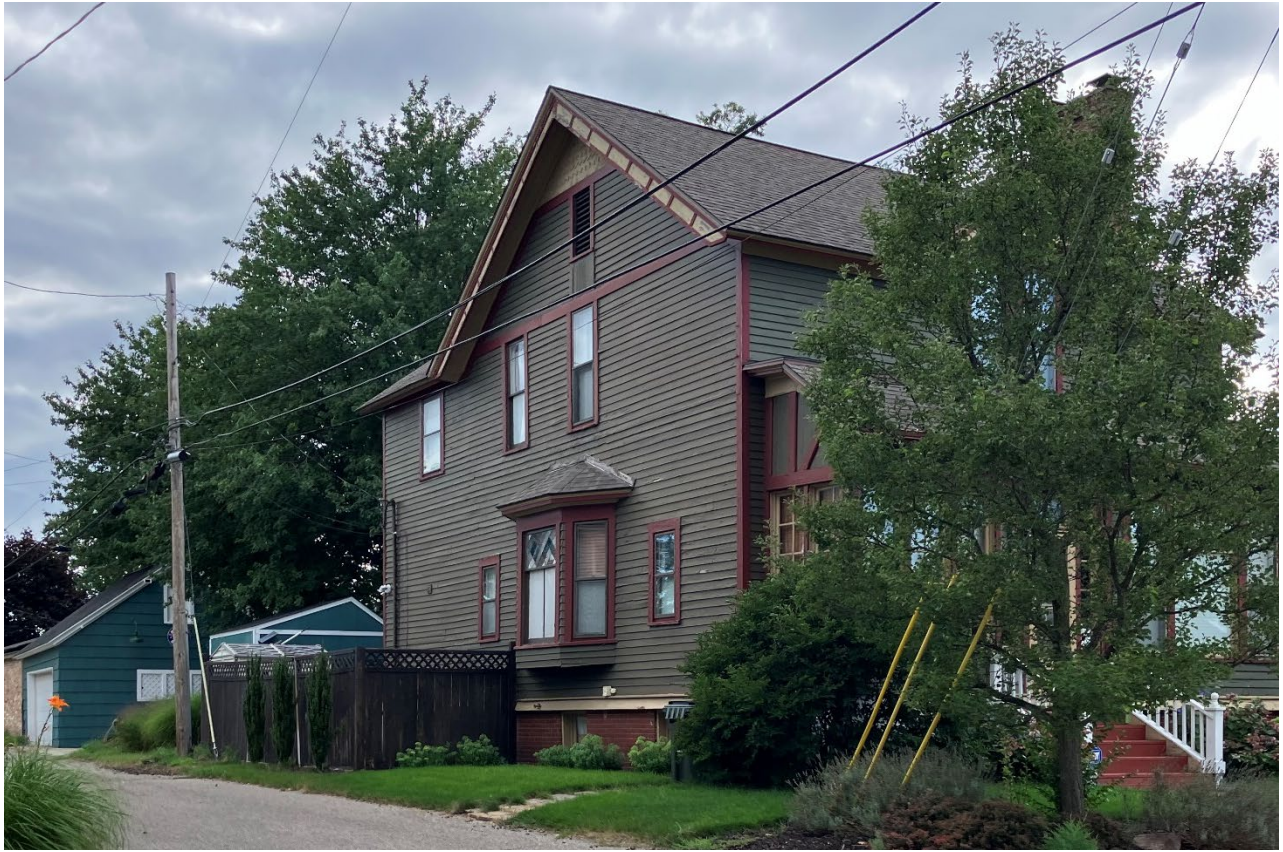
Three second-story windows on the south elevation proposed to be replaced.
