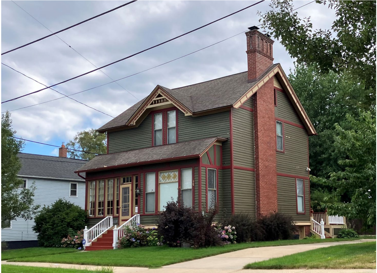
View of house from 5 th Street, looking south.
