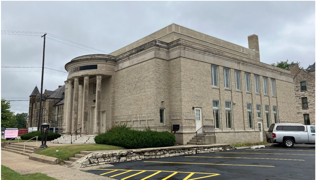
View of the south (front) and east (side) elevations from W. Muskegon Avenue.
