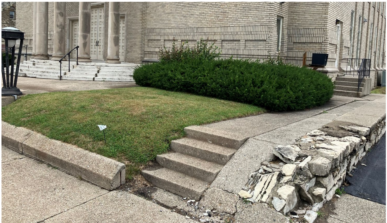
View of the proposed ramp location where it will connect to the sidewalk to the left of the stairs.
