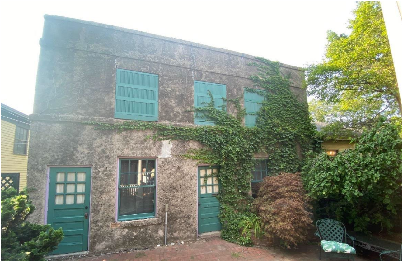
View of wall facing the main house, looking northwest.
