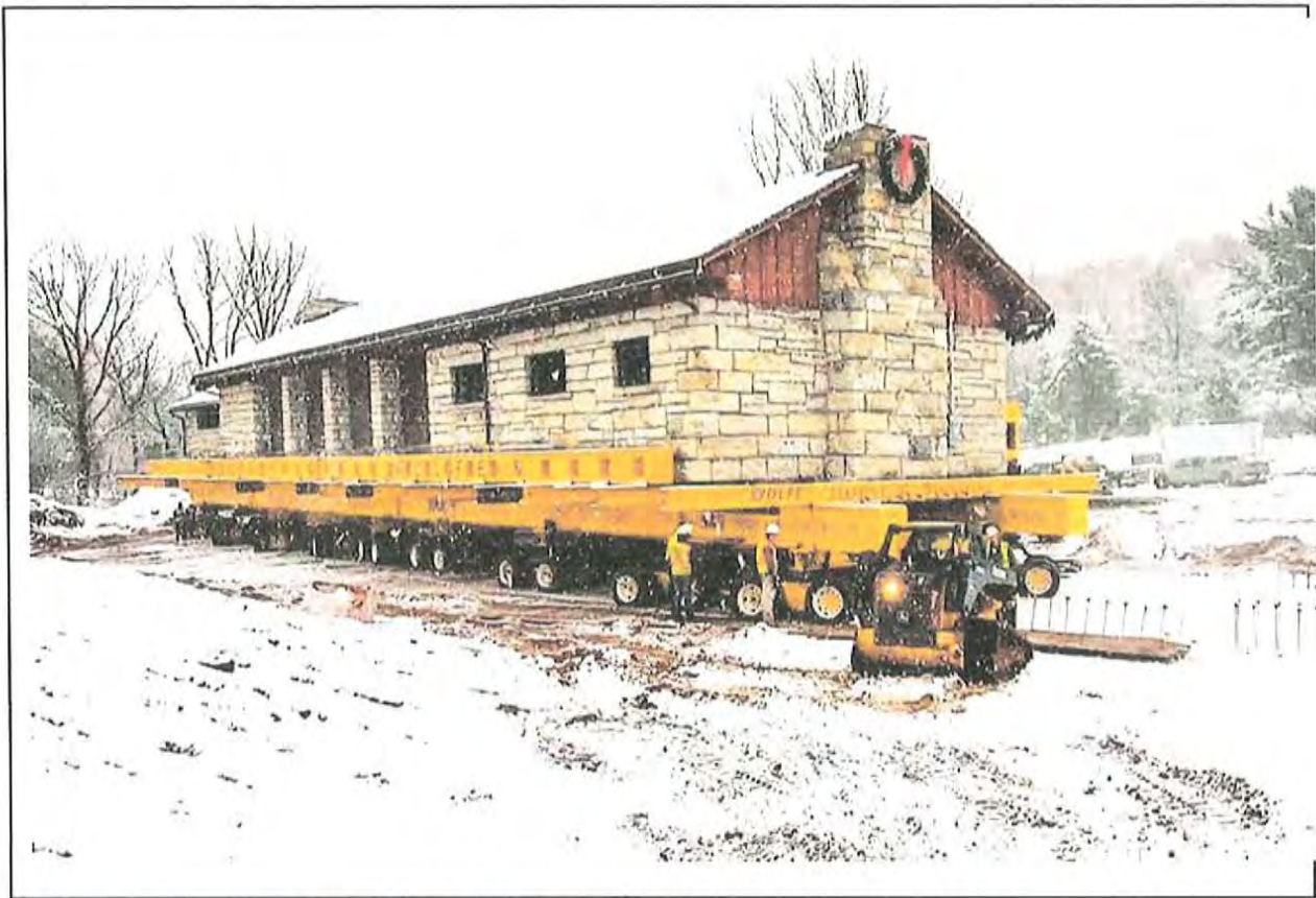
The Buckingham SmartSteer® System steers a stone park pavilion around a corner and into place over its new foundation.
