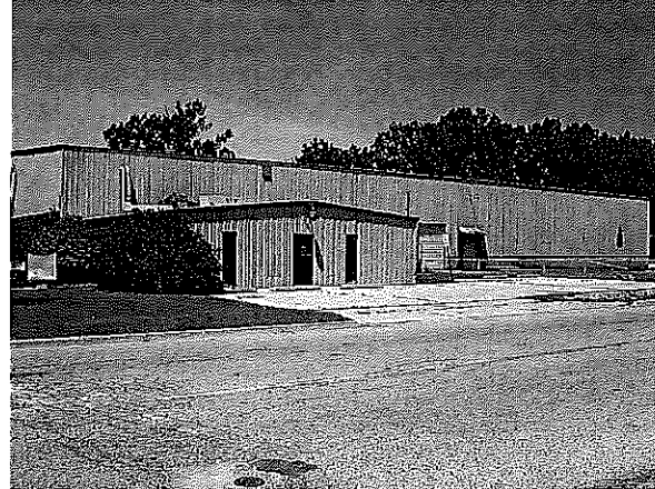
Side of the building from across Sundolphin.
