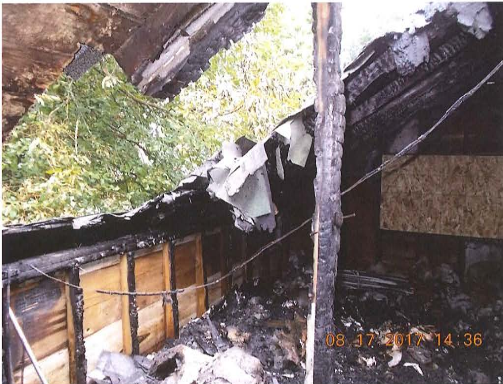
Top of Stairway looking to rear of home
