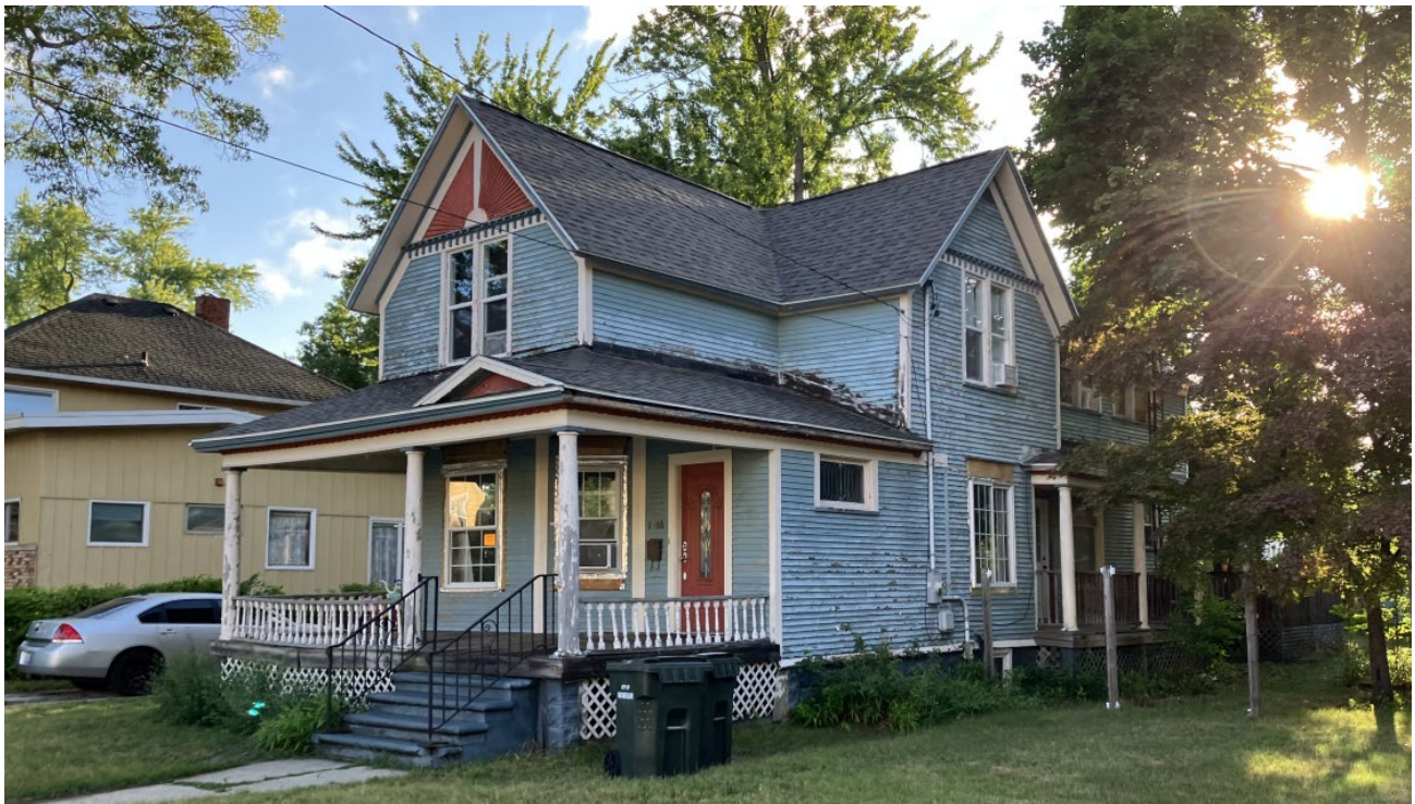
View of west (front) and south elevations from Peck Street, looking northeast. Unapproved replacement windows visible on first-story.
