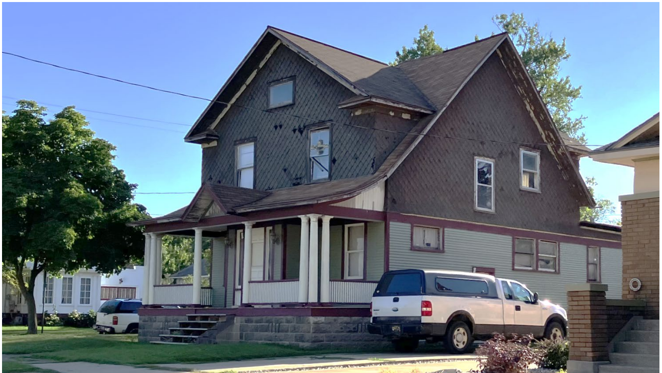
View of east and north elevations from Clinton Street. Larger second-story window on north elevation (currently only a storm window) is proposed to be replaced. The pair of adjacent, first-story windows on the north elevation are proposed to be replaced with a single window filling the windows' original openings.
