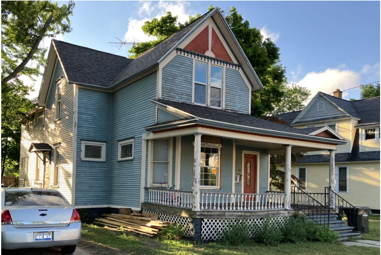
View of north and west elevations from Peck Street. Unapproved replacement window visible on front porch.
