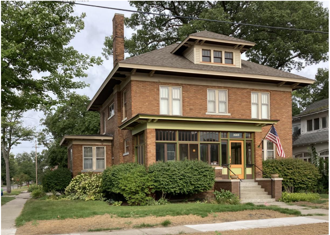
View of house from Peck Street looking west.
