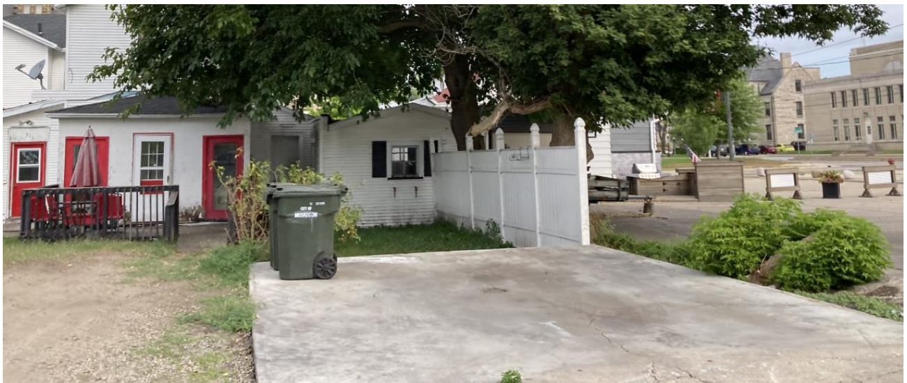
View of remaining concrete pad looking north from alley (August 2021)
