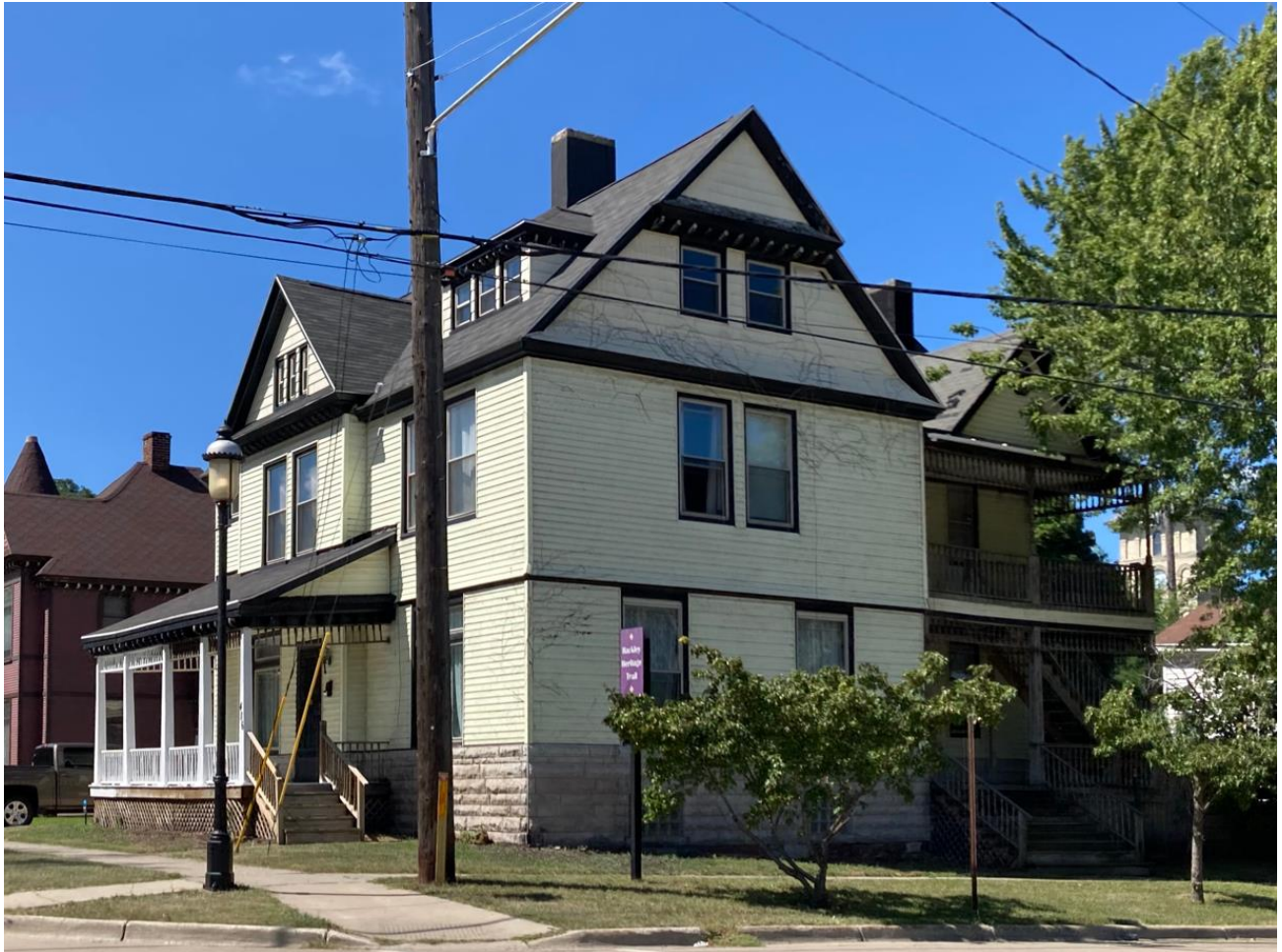
View of house from 5 th Street looking west, with side porch visible at right.
