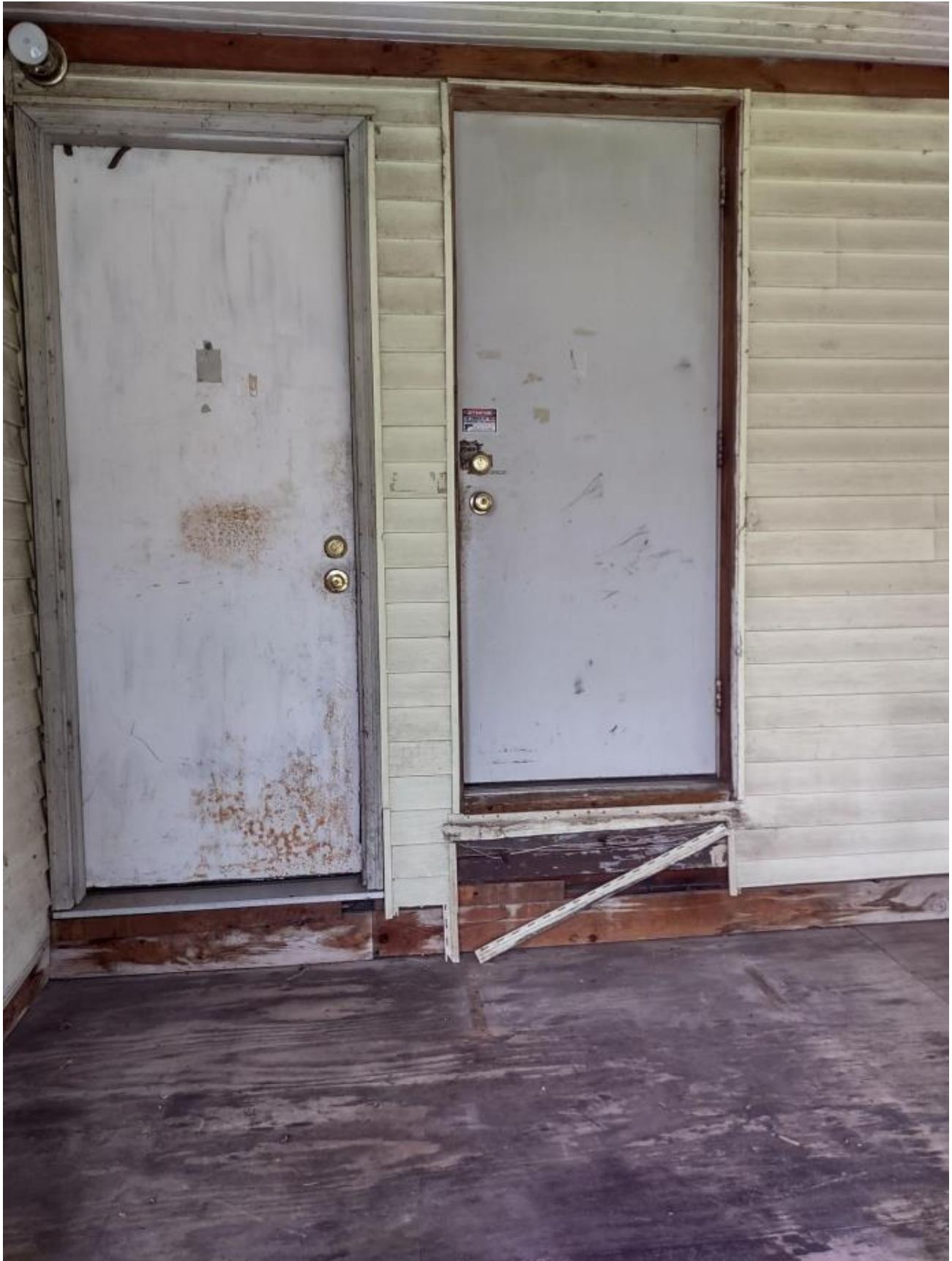
Exterior doors on the upper porch. The right door is proposed to be removed and resided to match the rest of the house. The left door is proposed to be replaced with a more energy efficient door.
