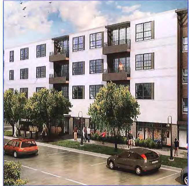
New Construction of a 4 to 5-story Mixed-use Building with Rooftop Lounge
