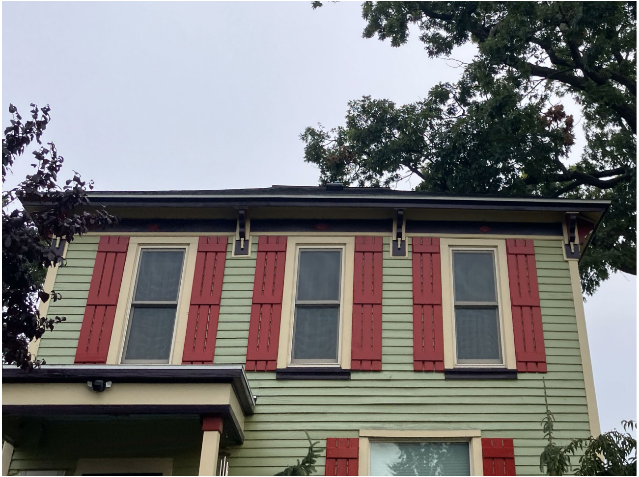
Detail view of shutters.
