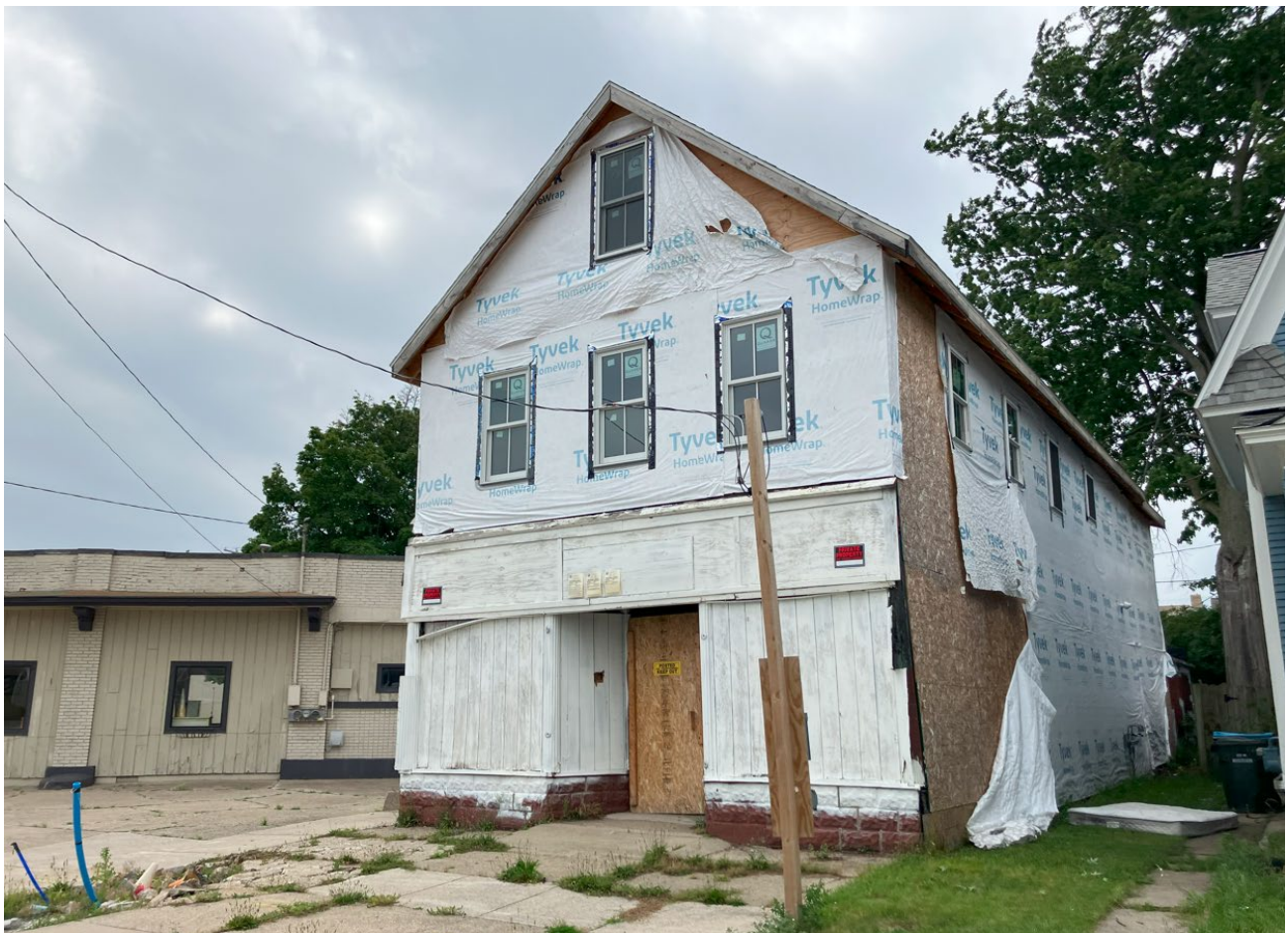
View of building from Houston Avenue, looking west.
