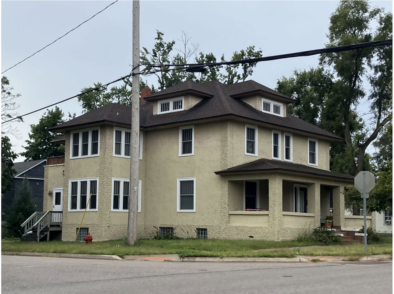
View of building from W. Muskegon Avenue, looking south. Side porch stairs visible at left.
