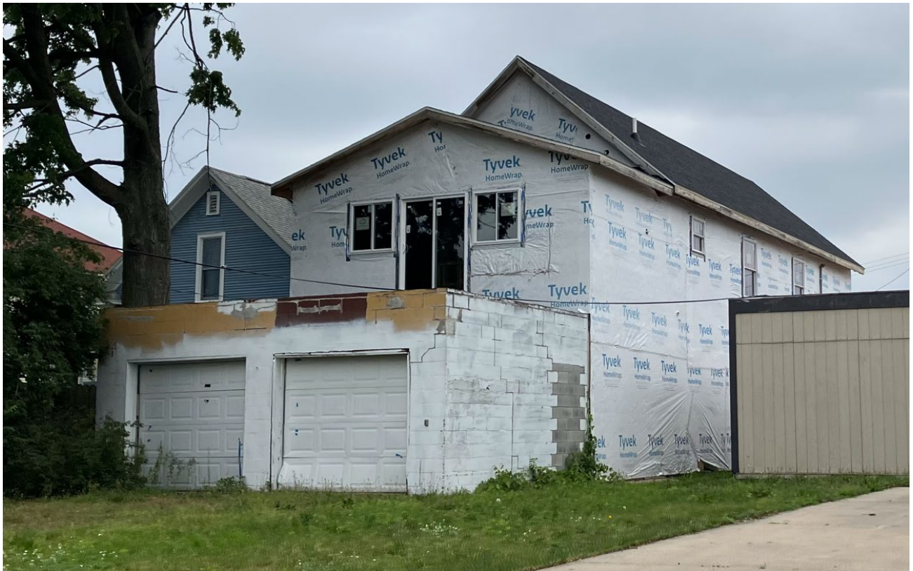
View from rear alley, looking east.
