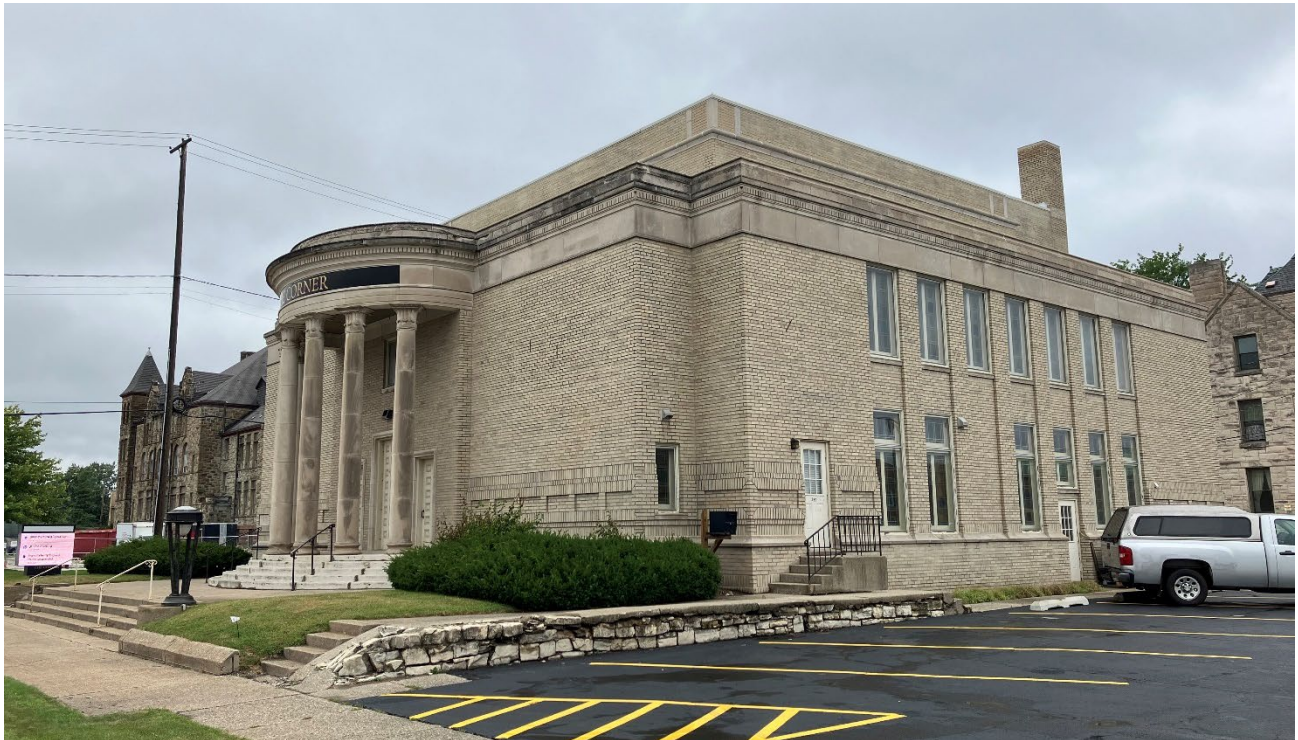
View of the south (front) and east (side) elevations from W. Muskegon Avenue.
