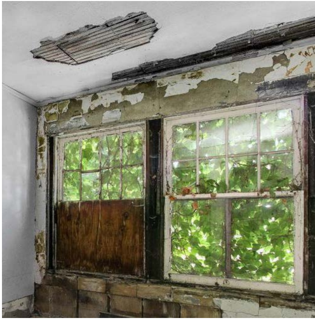
Existing window mullion pattern
