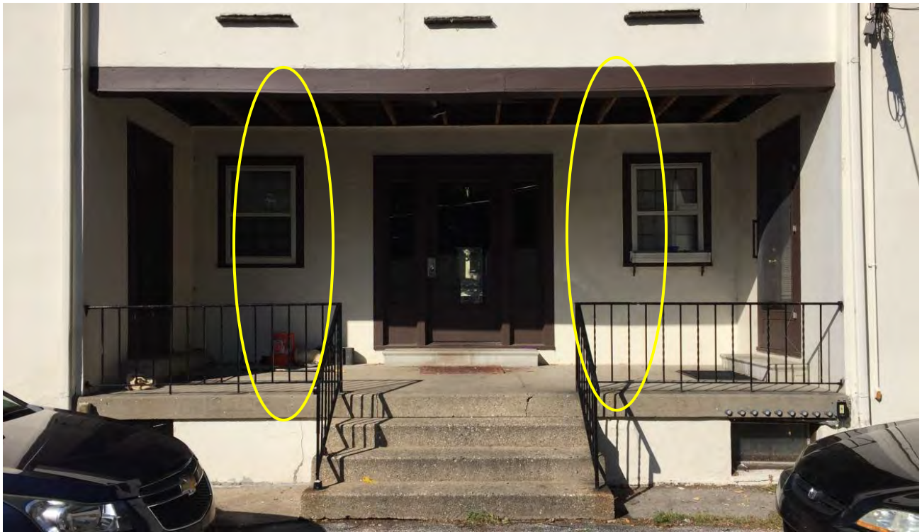
Rear balcony highlighting proposed location of jack posts
