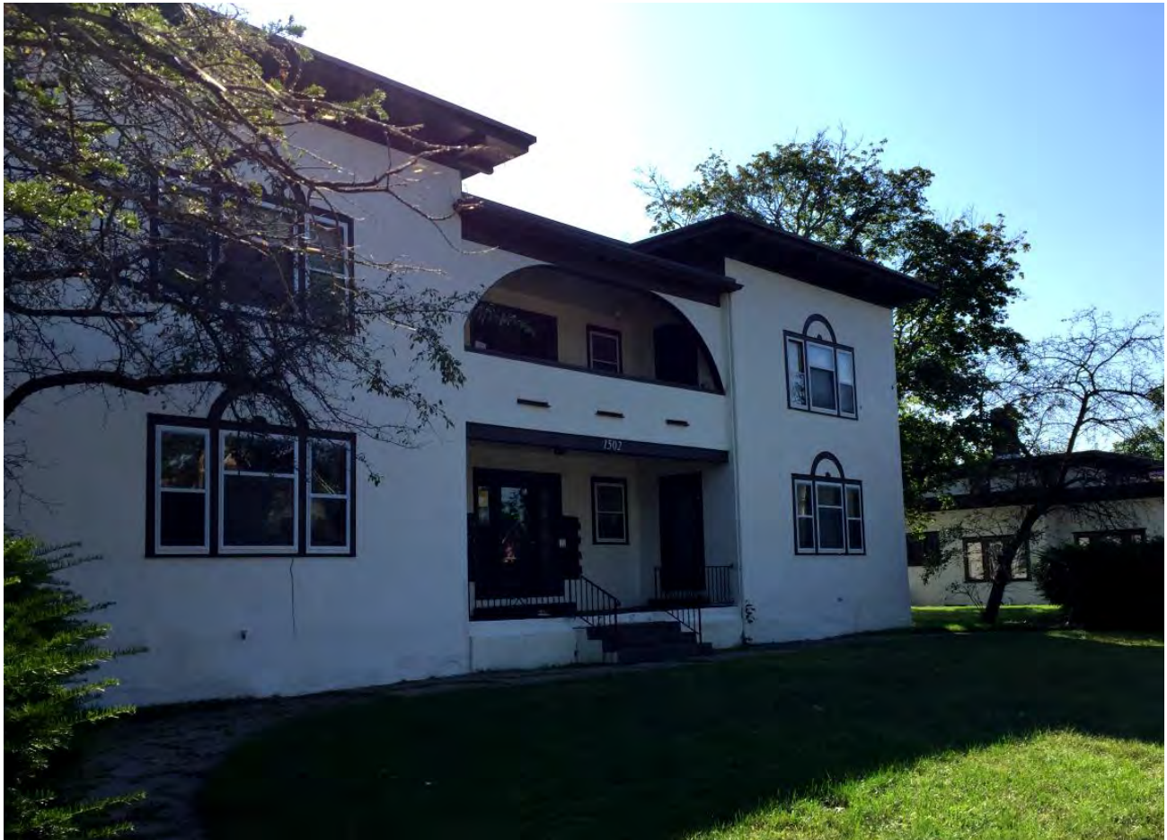
View of structure from Peck Street
