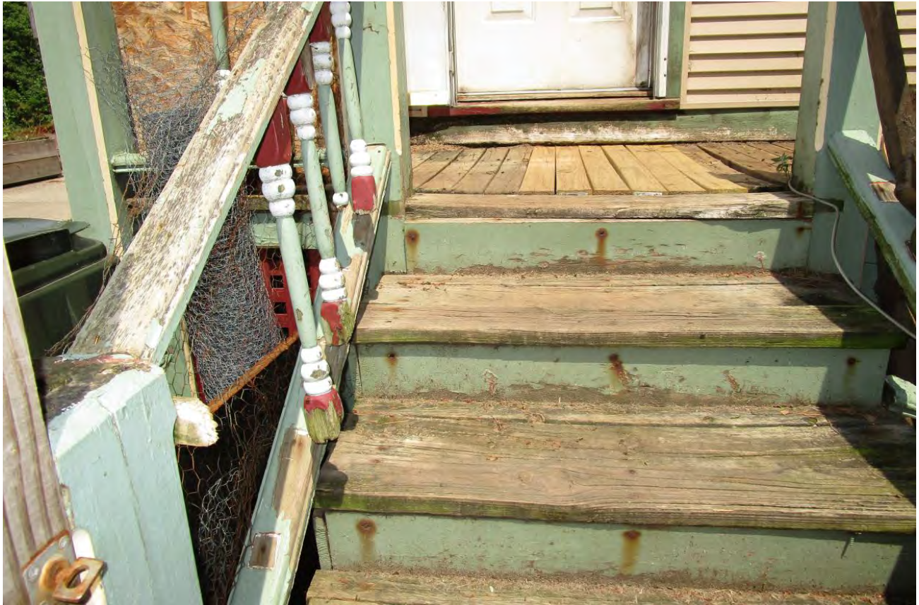
Rear porch stairs
