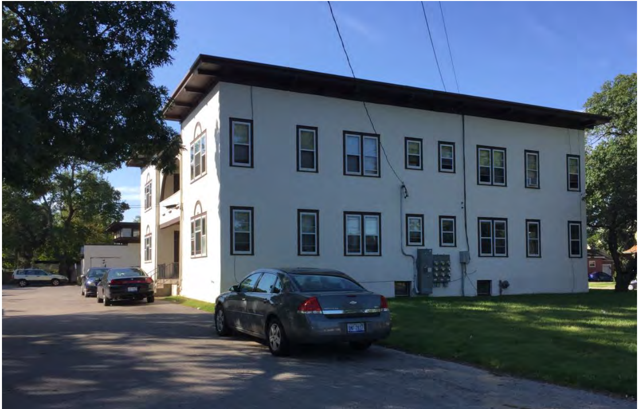
View of rear balcony from E. Grand Avenue
