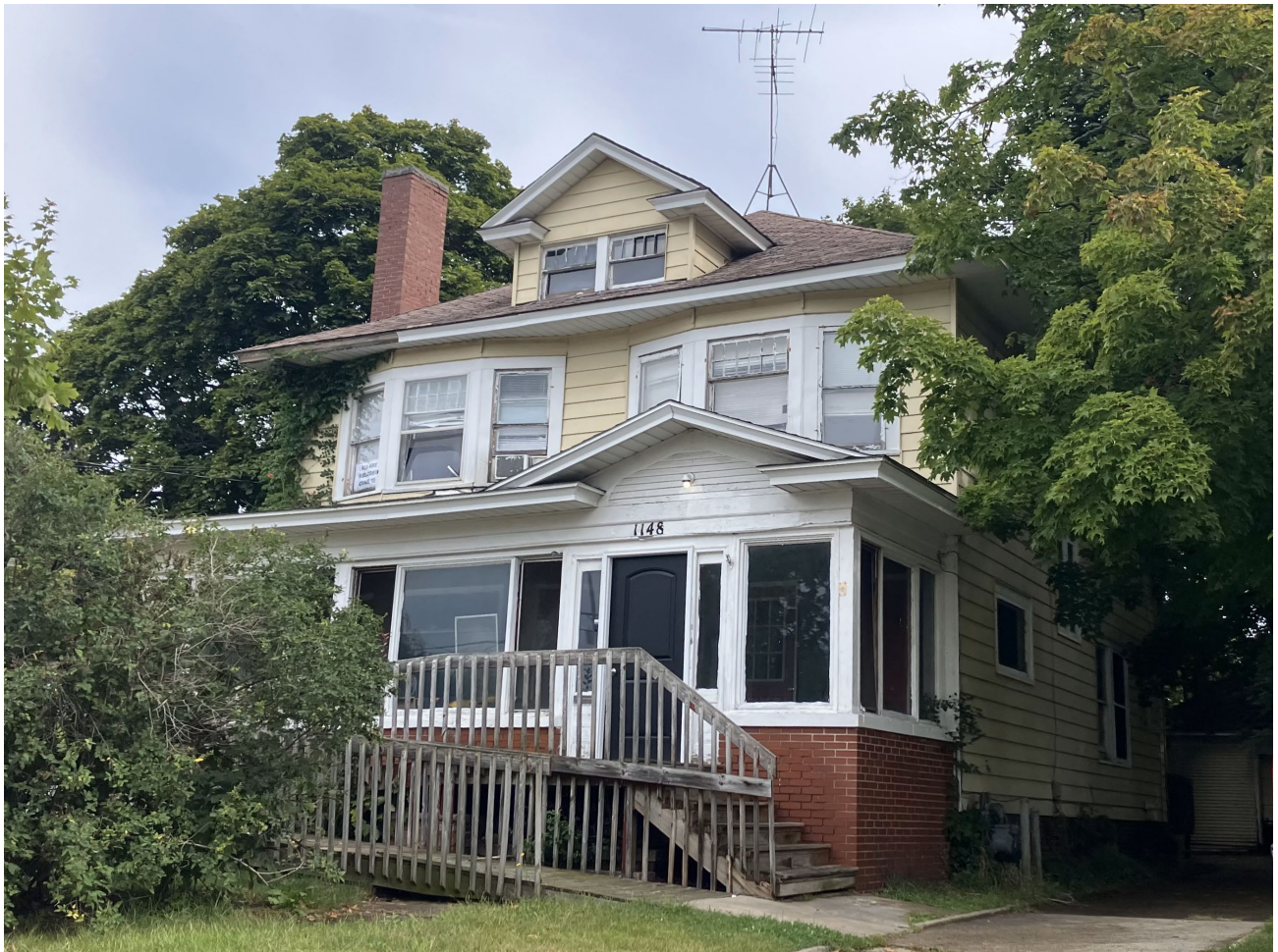
View of building from Terrace Street, looking north.
