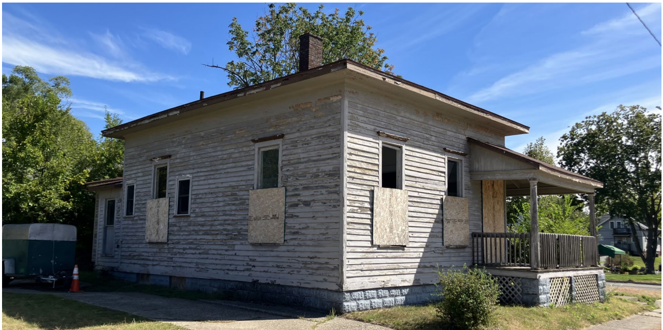
View from 6 th Street, looking east.
