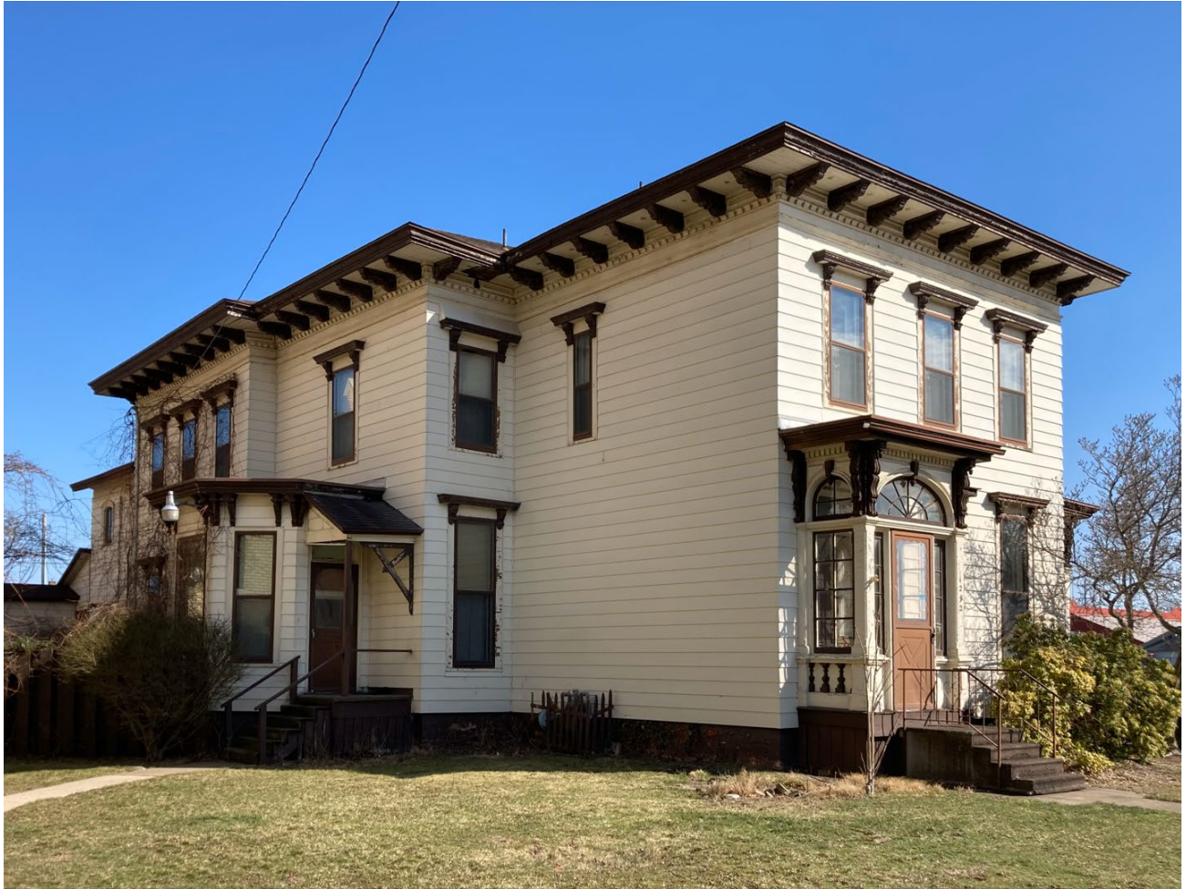
View of the house at 1292 Jefferson Street (photo from March 2021).
