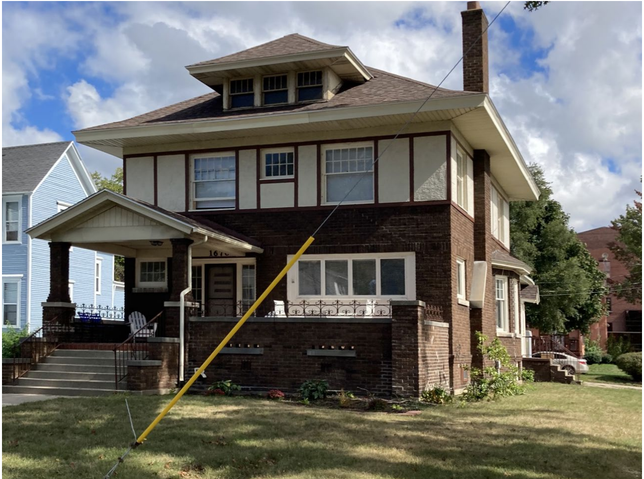
View of house from Peck Street, second floor windows visible would be replaced
