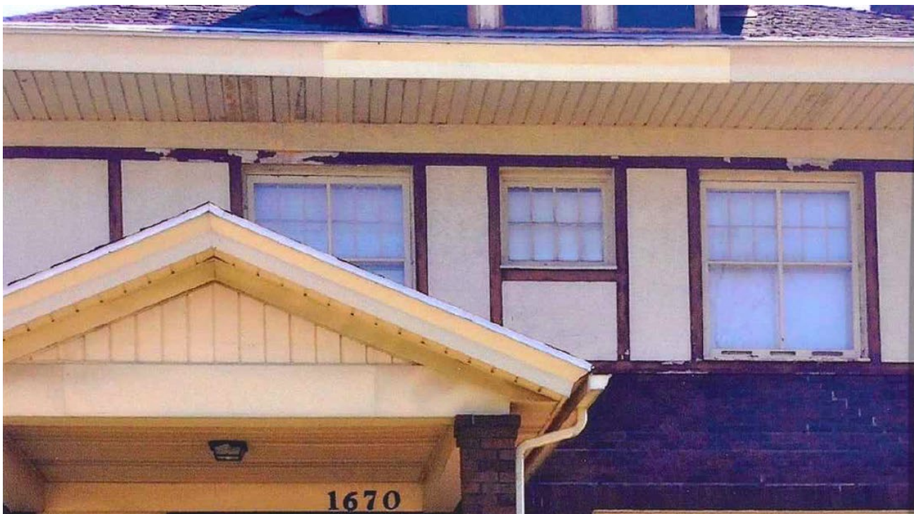
Windows on the west façade (facing Peck) with large storm windows installed
