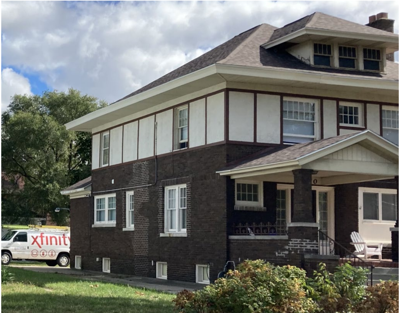
North facade viewed from Peck Street, second floor windows visible would be replaced
