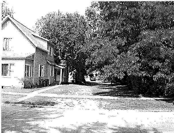
View looking northwest at 236 Monroe.
