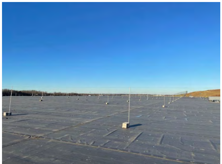
Typical pole layout supporting grids on a large warehouse roof. No roof penetration.
