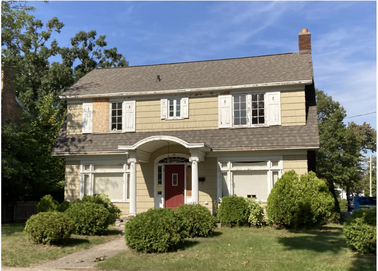
View of south elevation from W. Grand Avenue looking north. Four second story windows proposed to be replaced.
