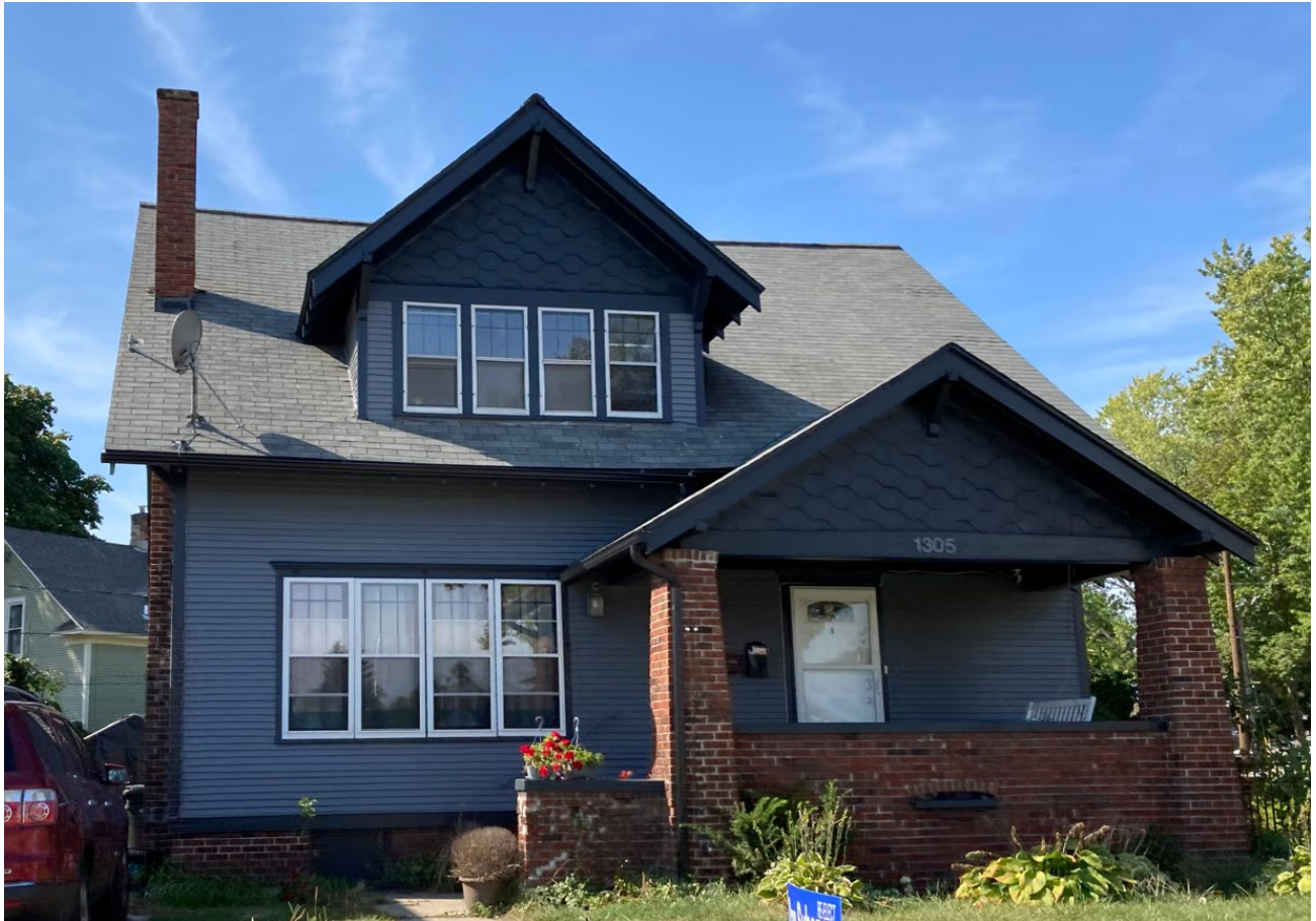
View looking west from Jefferson Street.
