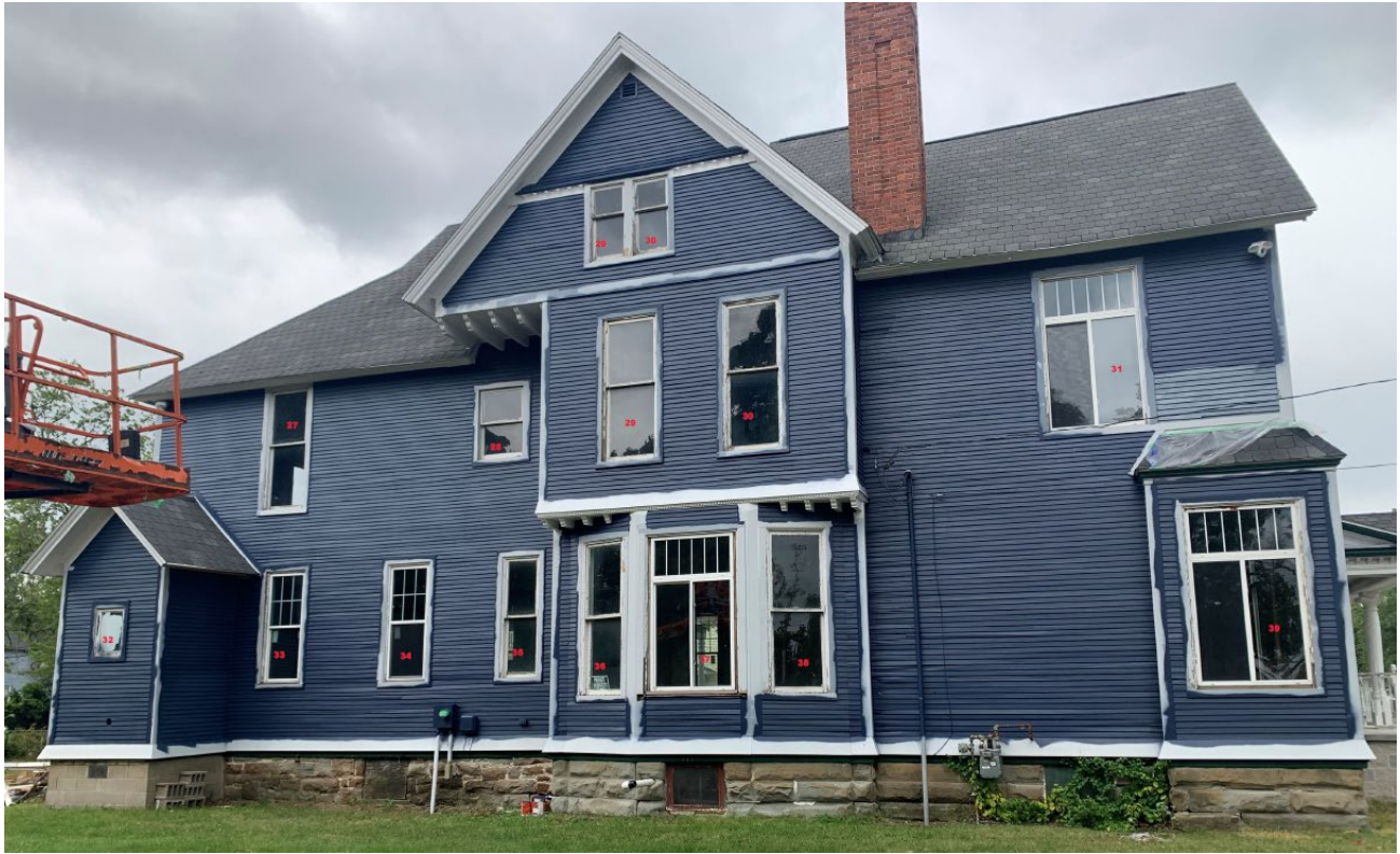
West elevation with proposed replacement windows noted.
