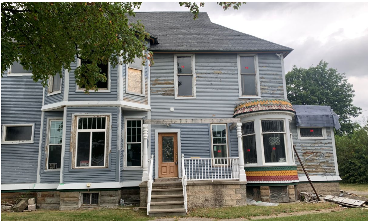
Additional view of east elevation with proposed replacement windows noted. East and north porch visible (rear porch has already been removed).
