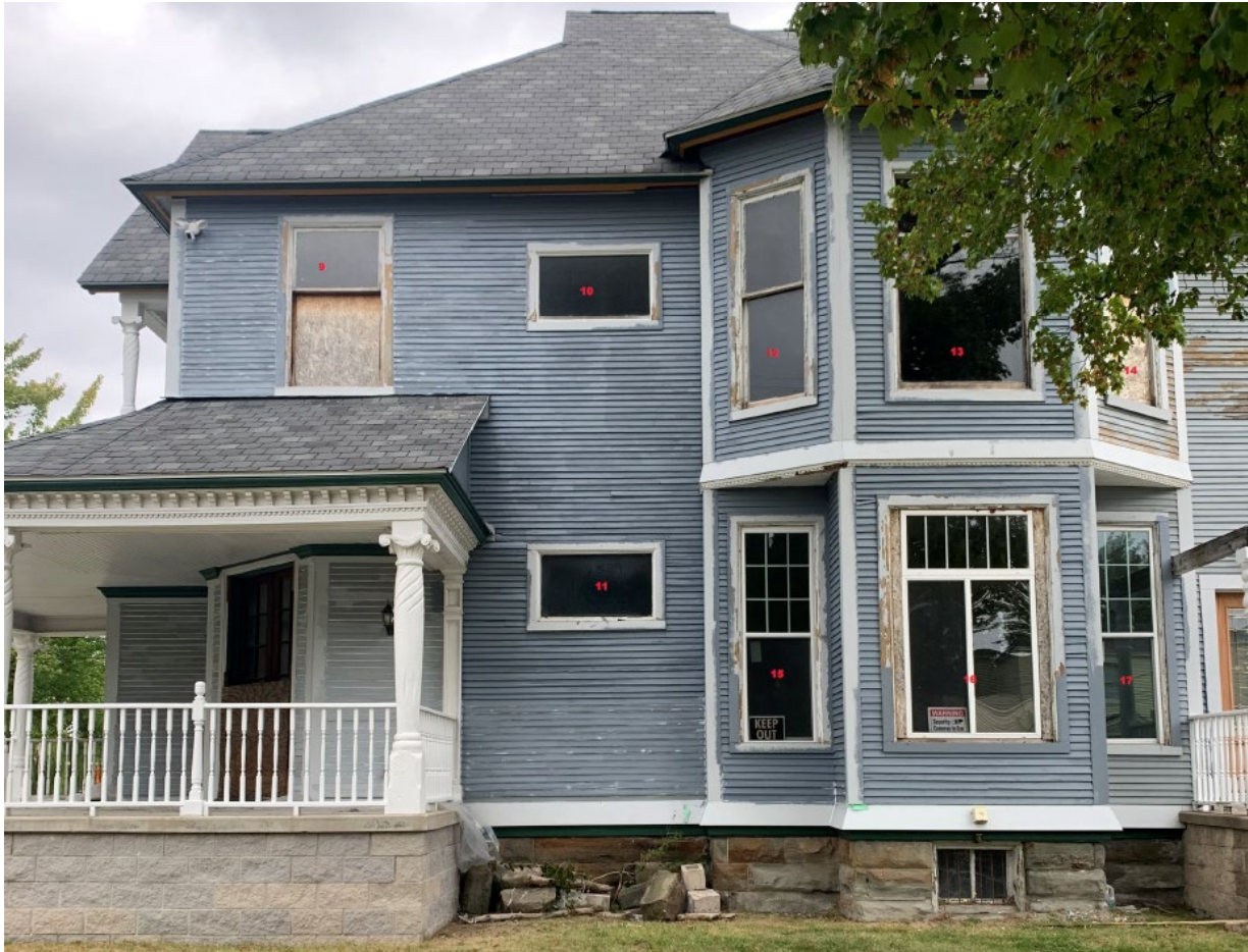
East elevation with proposed replacement windows noted.
