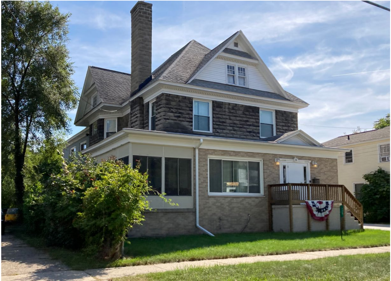
View of house from Delaware Avenue, looking south.
