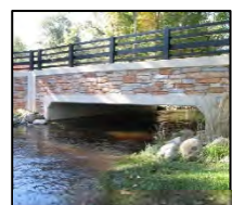
Figure 4: Three-sided box bridge
