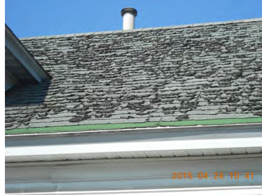
Roof up close.
