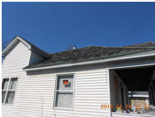
East side of structure/roof.
