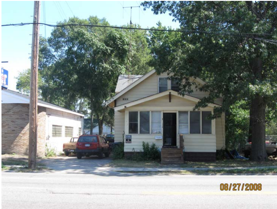
Subject home located at 1338 S. Getty Street.
