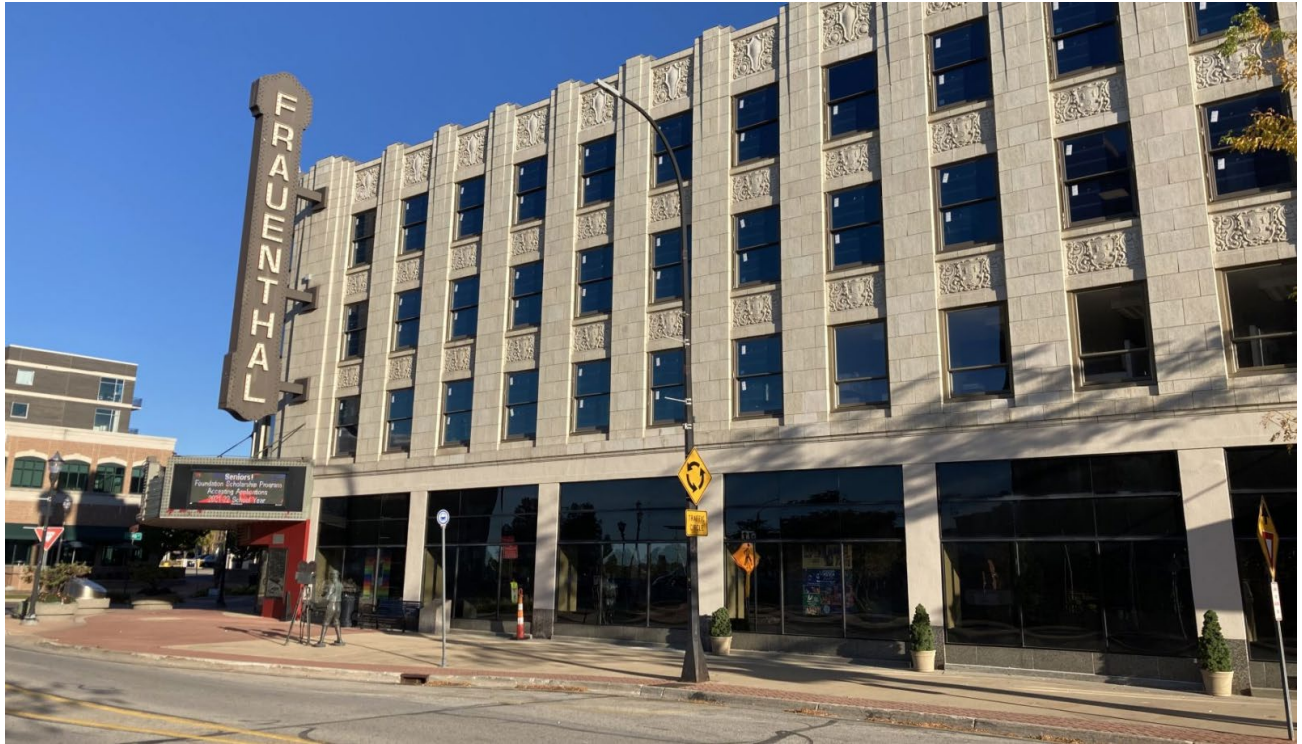
View of structure from W. Western Avenue with previous windows visible at right
