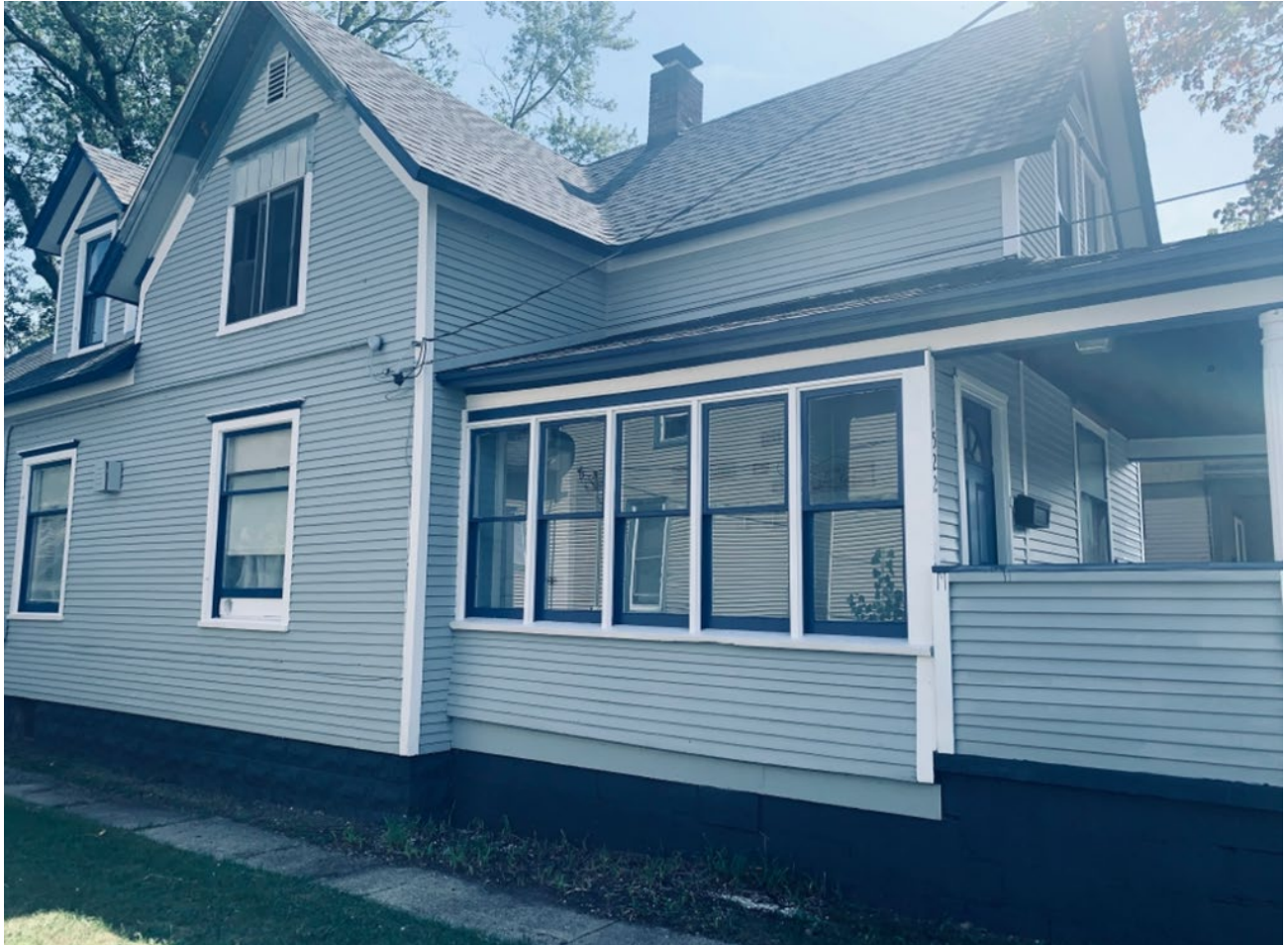
View of house from side yard, new garage out of view at left
