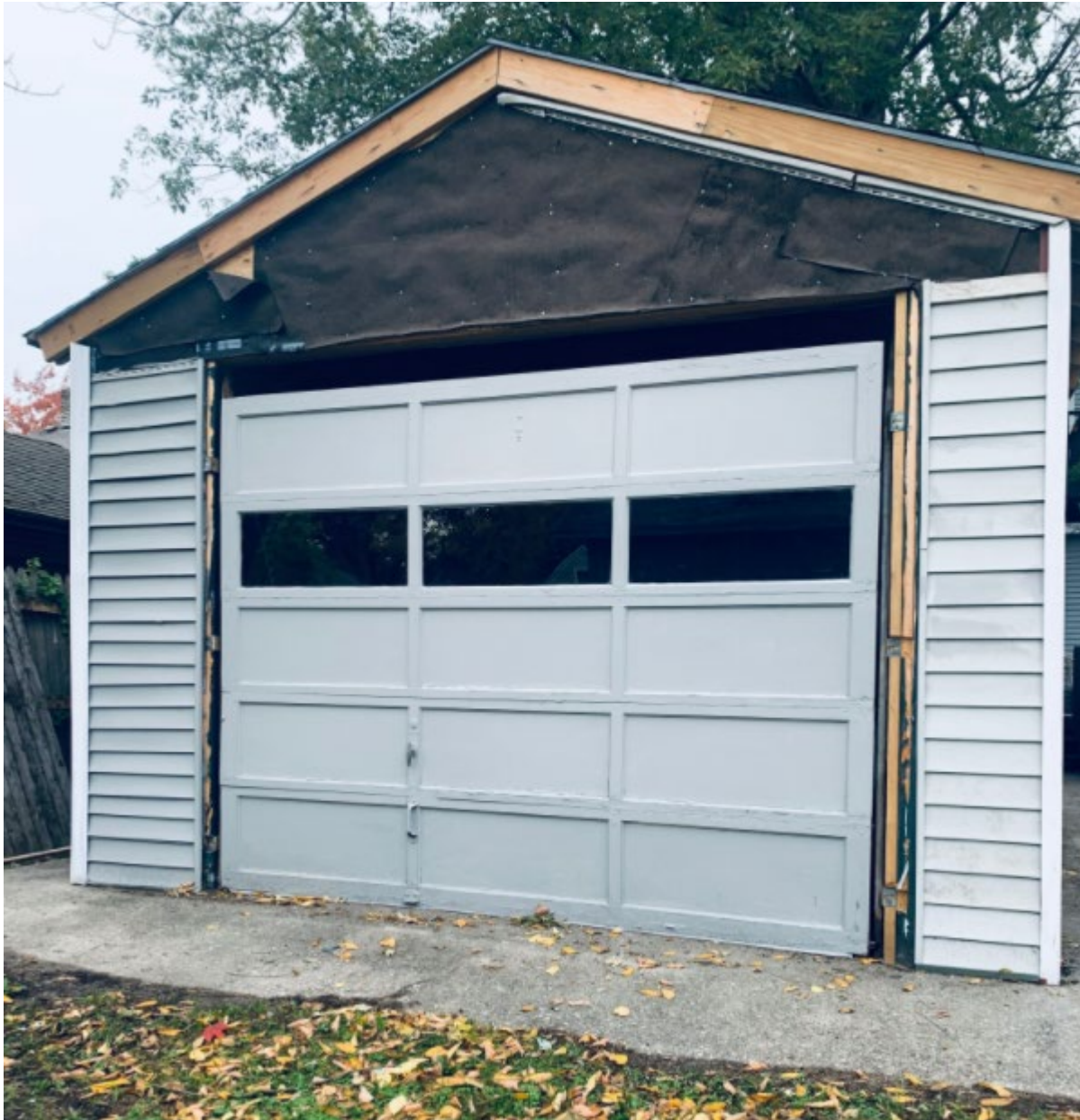
View of new garage from rear alley
