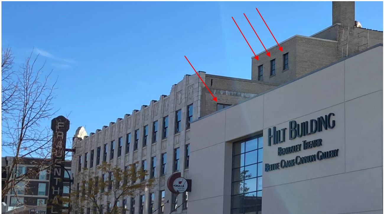
View showing three windows in elevator equipment room and one west-facing window
