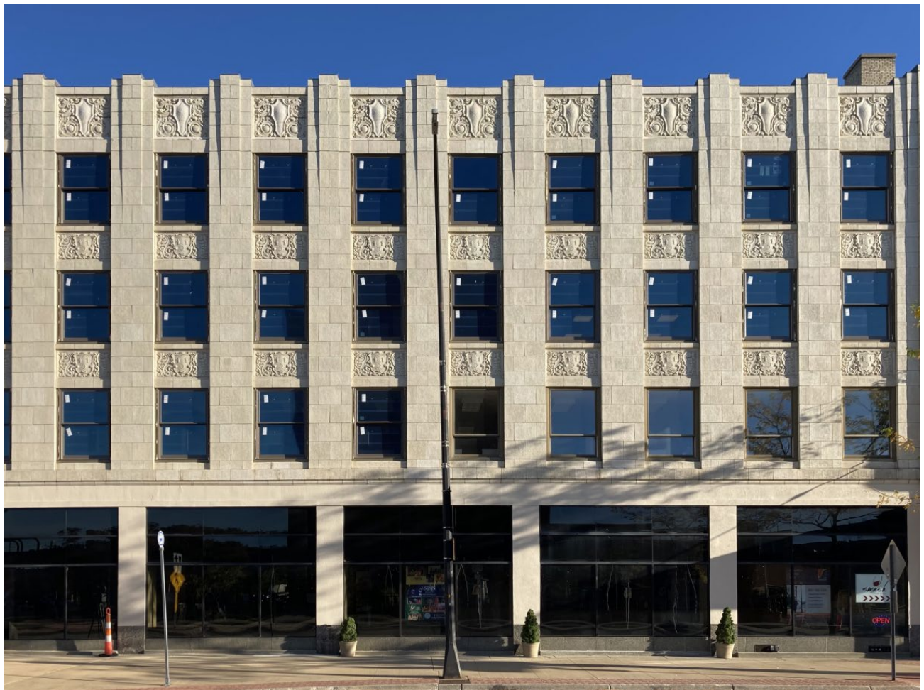
View of north façade showing design of new and existing windows
