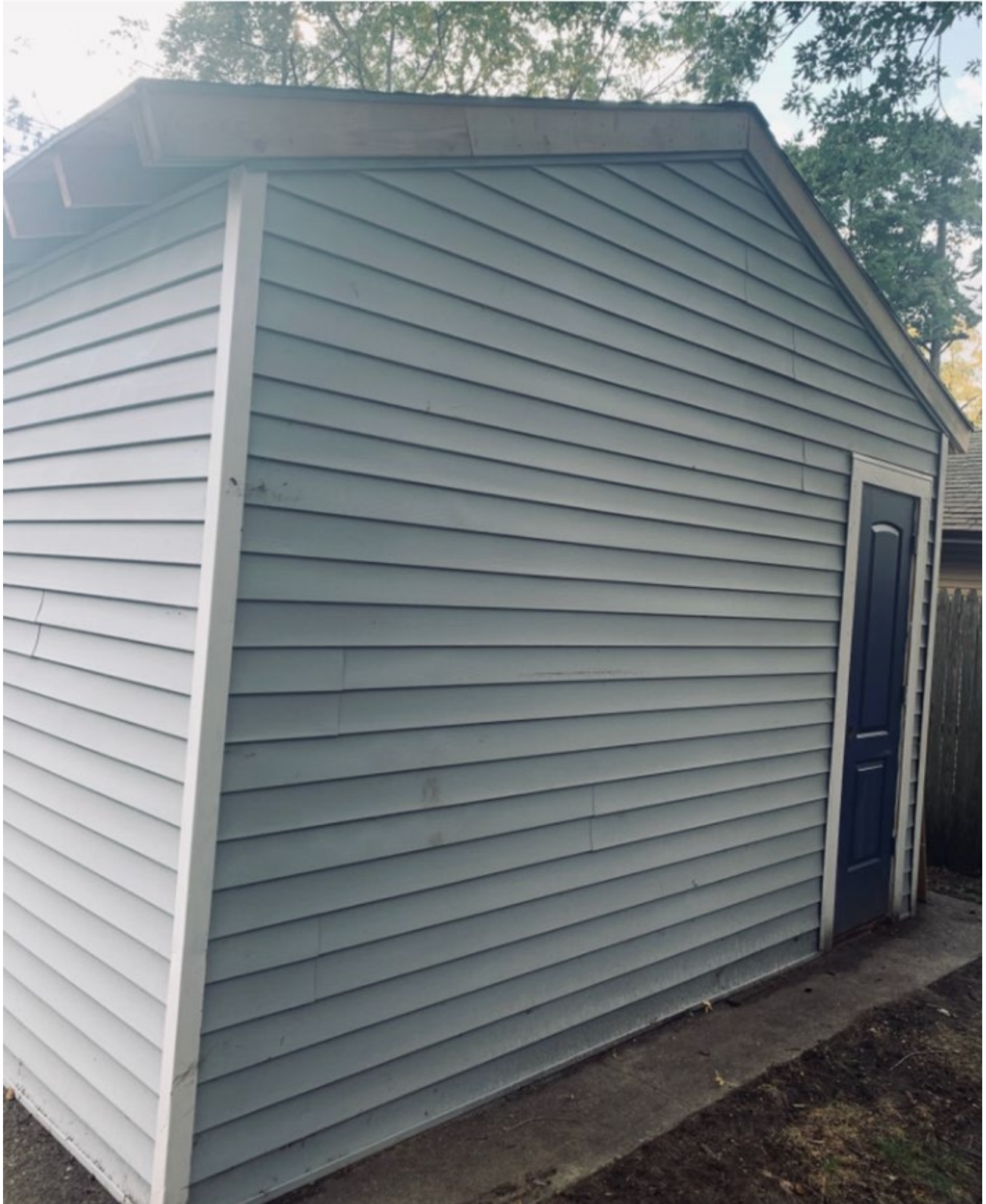
View of new garage from rear yard
