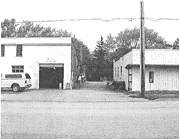
Alley looking north from E. Keating Ave.
