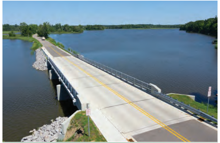
MARATHON ROAD BRIDGE
