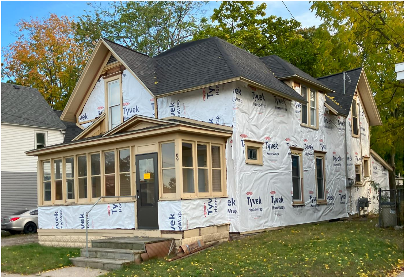
View of north (front) and west (side) elevations from Irwin Avenue.
