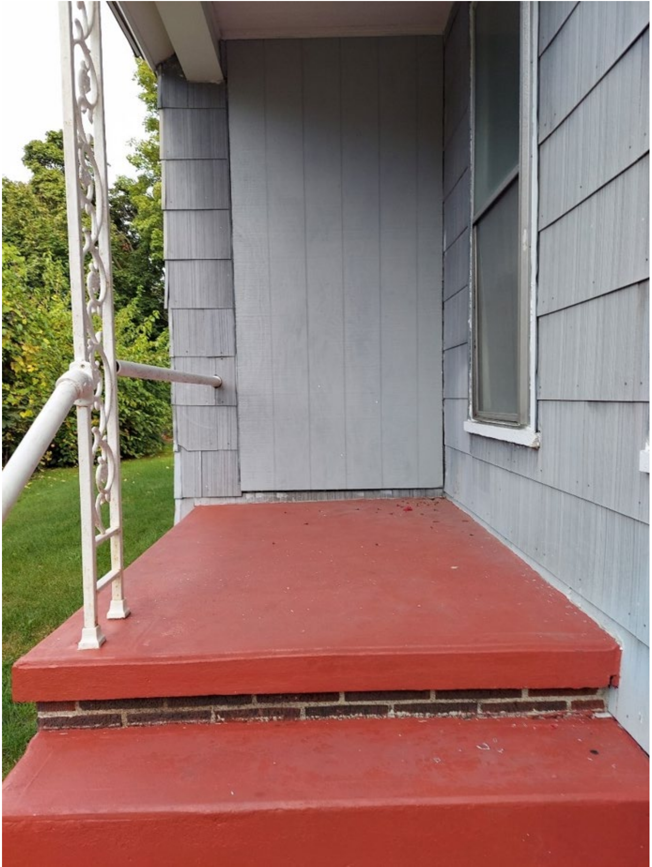
Current conditions: former location of entry door on side porch.
