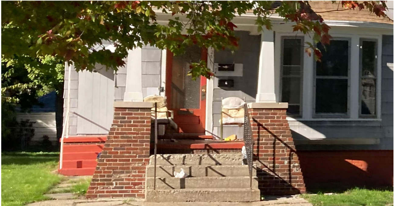
Existing front door to be refurbished is similar to appearance of former door on side porch.
