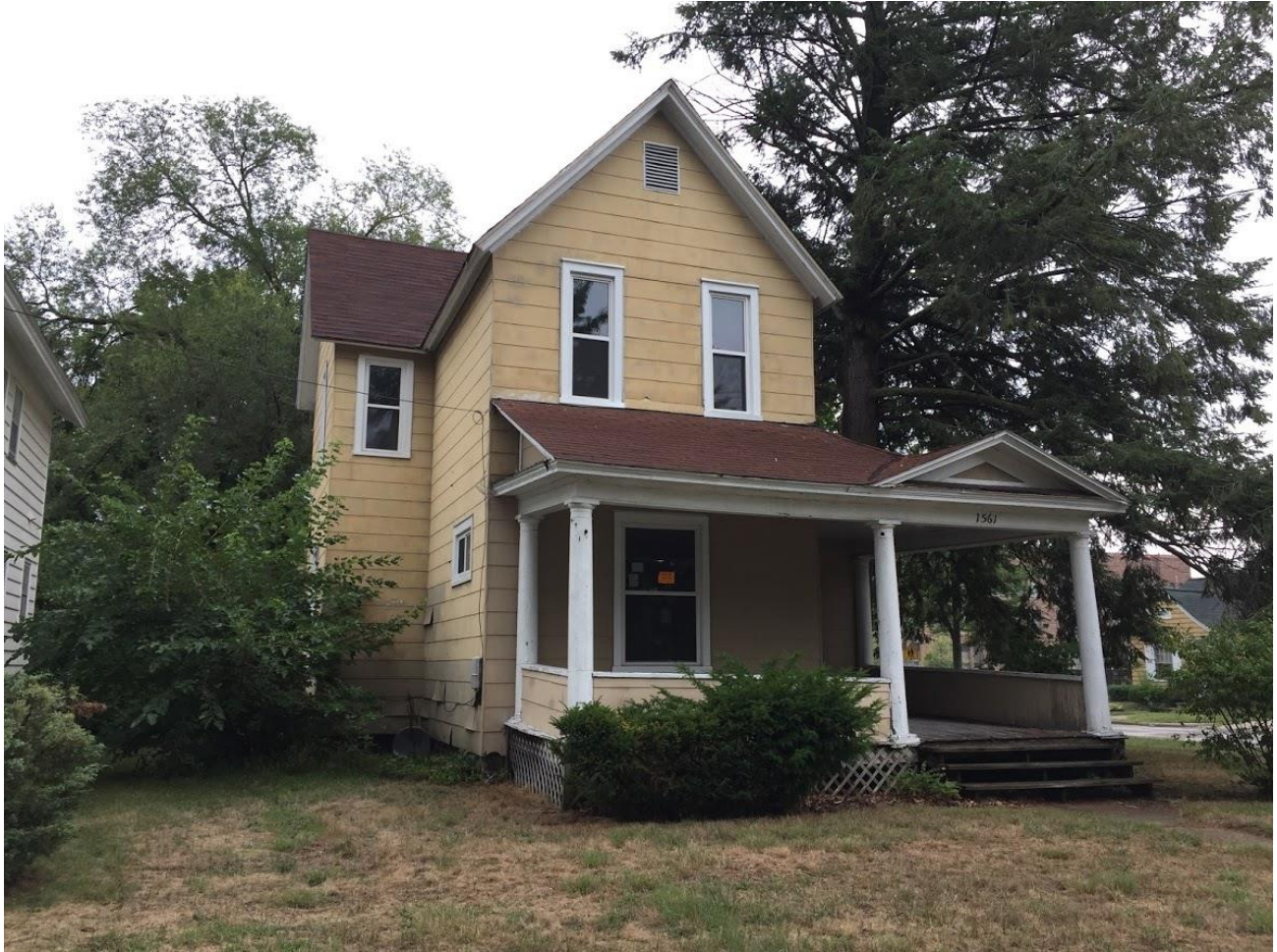
East façade with new vinyl windows
