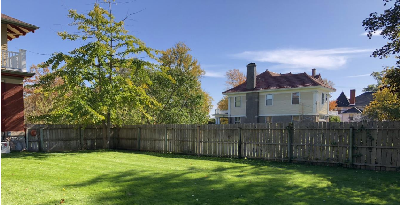
Wood fence to be replaced viewed from backyard
