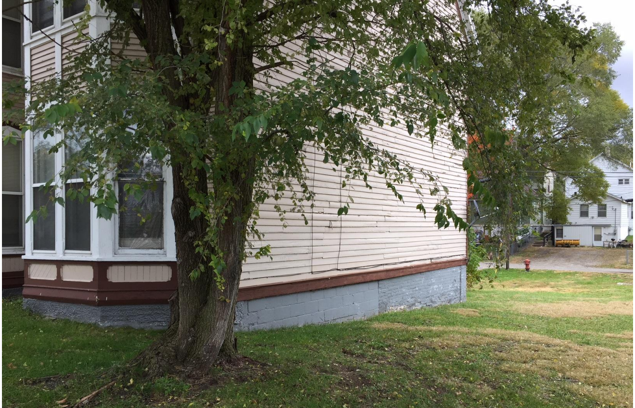
Southwest wall of structure
