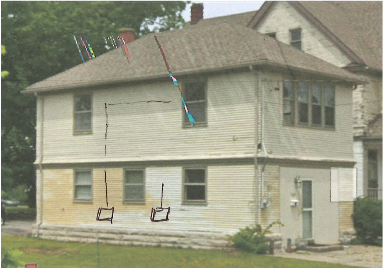
Proposed locations of mini-split HVAC units and route of conduit on south elevation.
