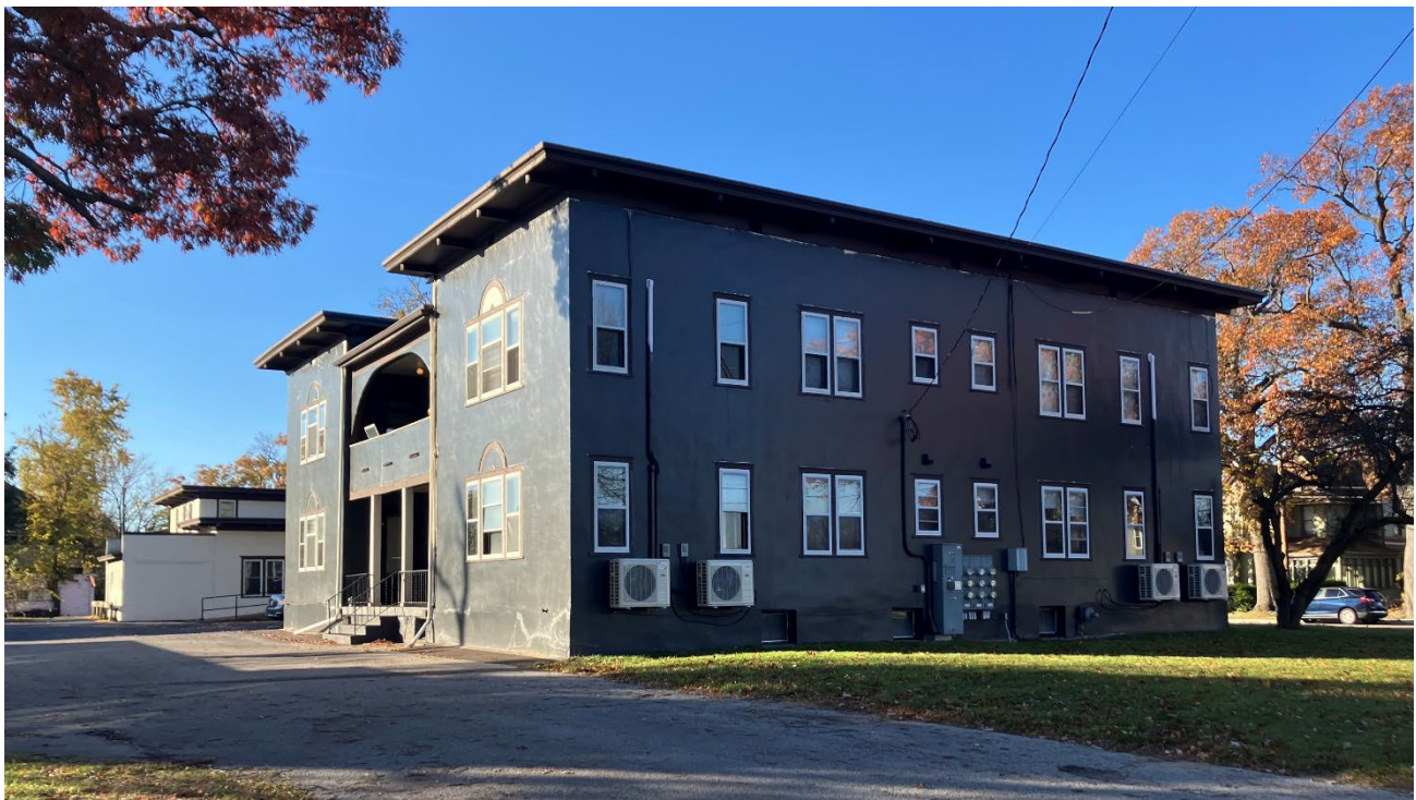
View of the north and east elevations from E. Grand Avenue, looking southwest.
