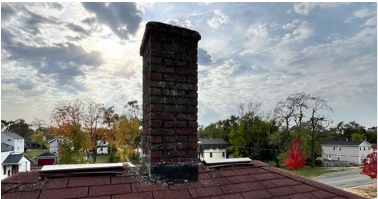
Detail view of chimney.
