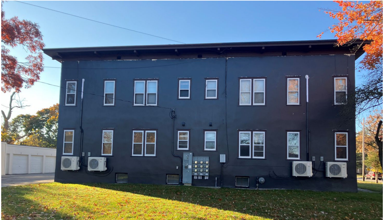
View of the north elevation from E. Grand Avenue, looking south.
