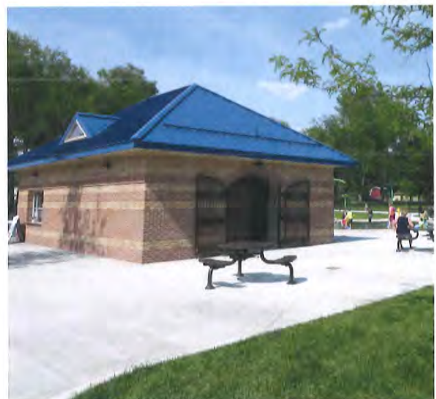
Georgetown Township, Rosewood Park Restroom
