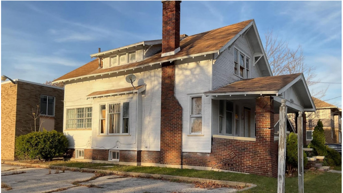
View of west elevation from Delaware Avenue (photo from November 2022).
