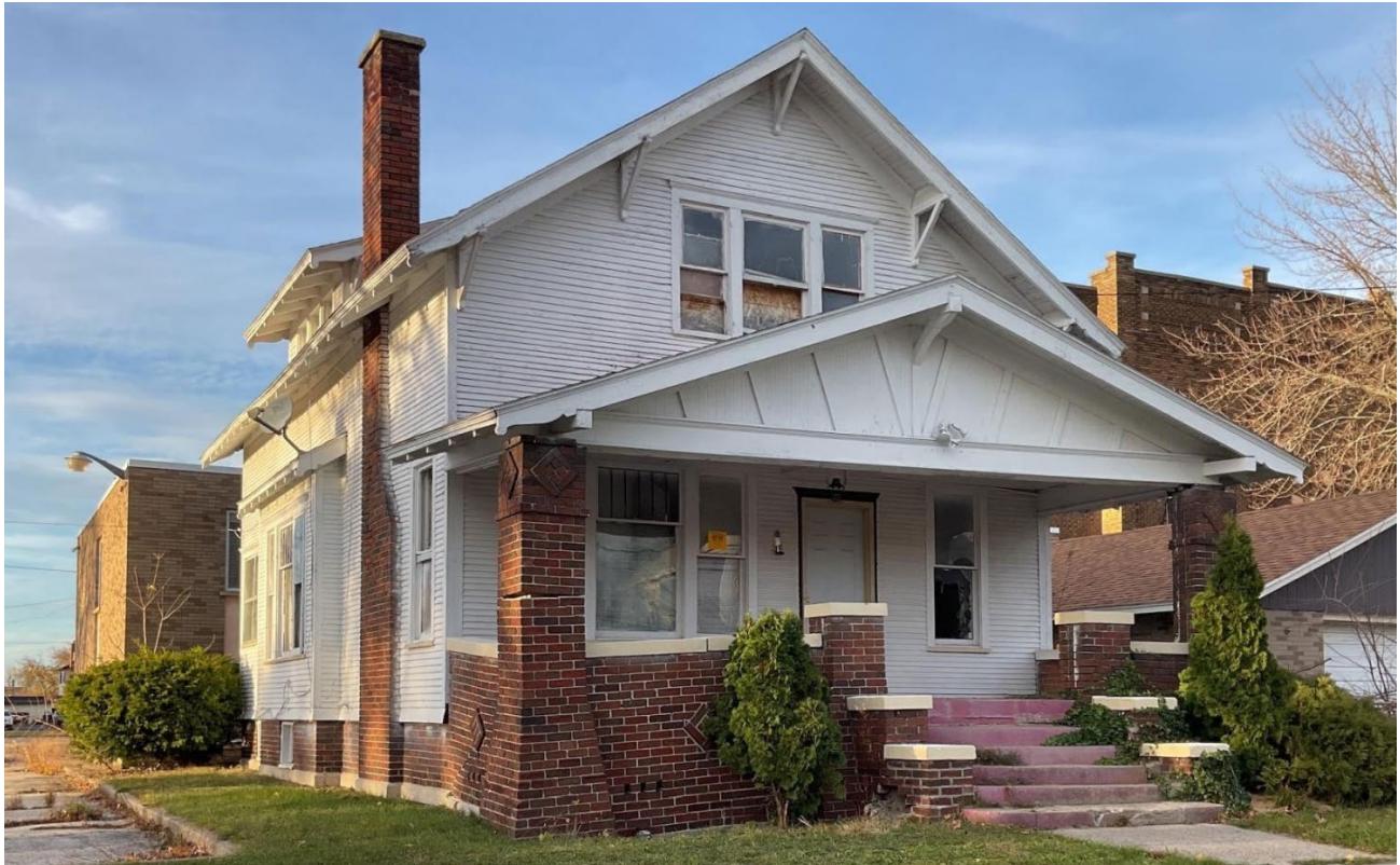
View of south elevation from Delaware Avenue (photo from November 2022).
