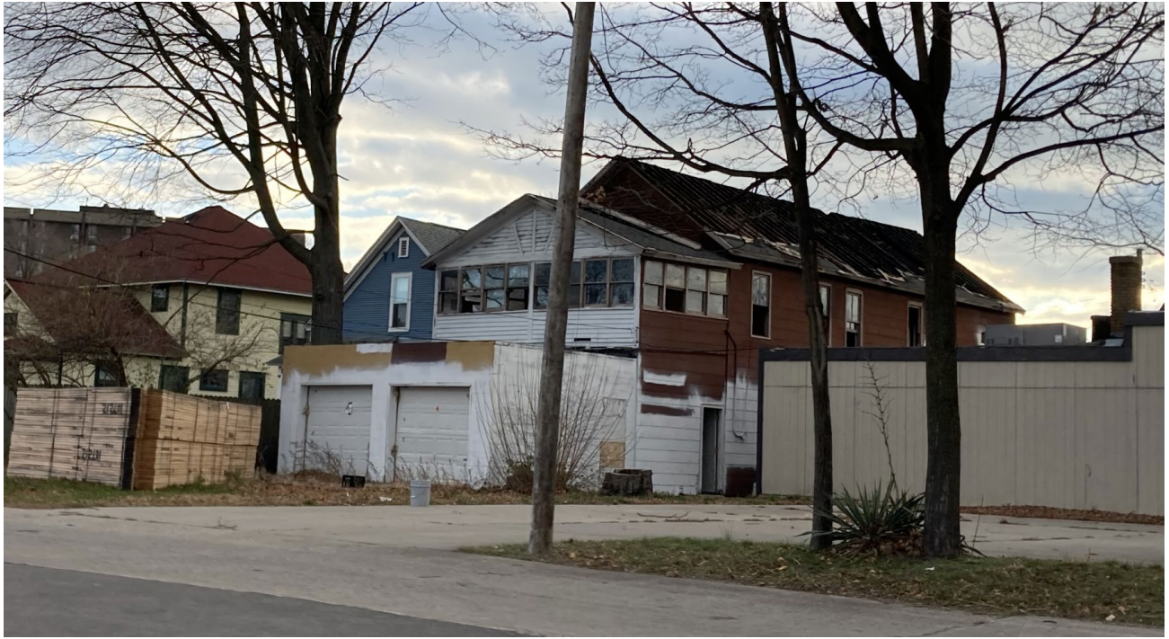
Rear of structure viewed from alley
