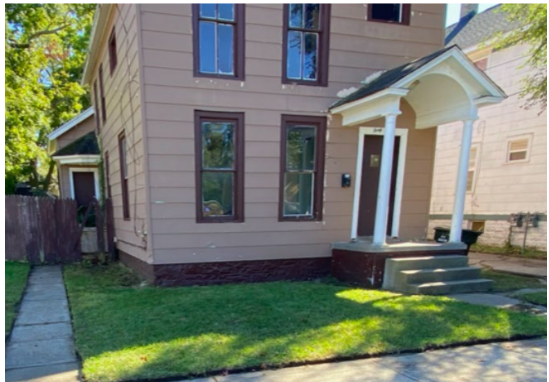
Existing front door and original windows
