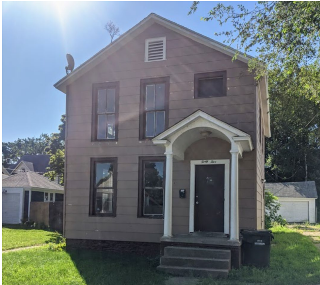
View of house before window replacement
