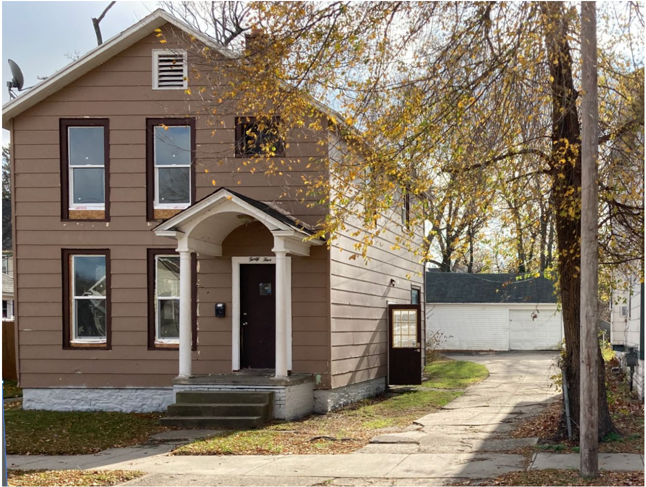
View showing detached garage with vinyl siding, alterations to window opening sizes, and the existing front door.
