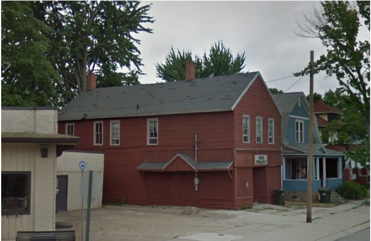
View of structure from 3 rd Street prior to the fire showing the roof and location of chimneys (photo from July 2018)
