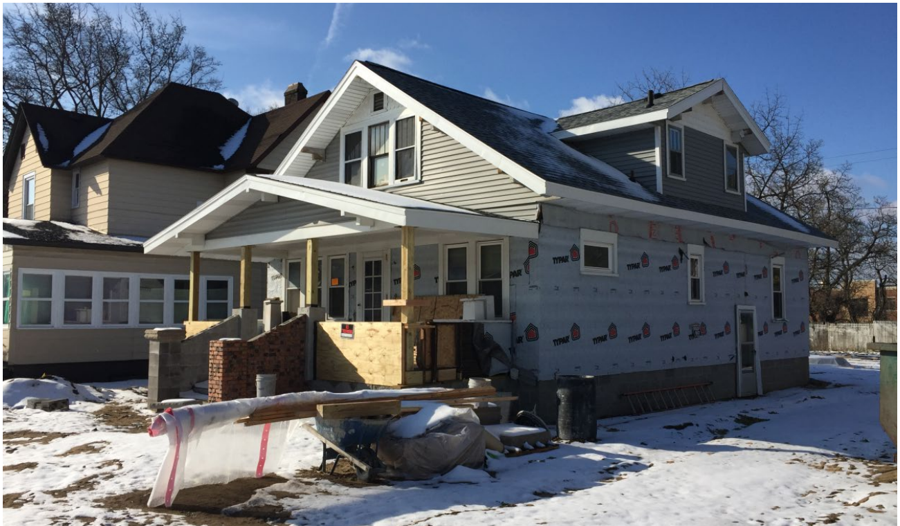
Door on northeast façade, visible at right, will be changed
