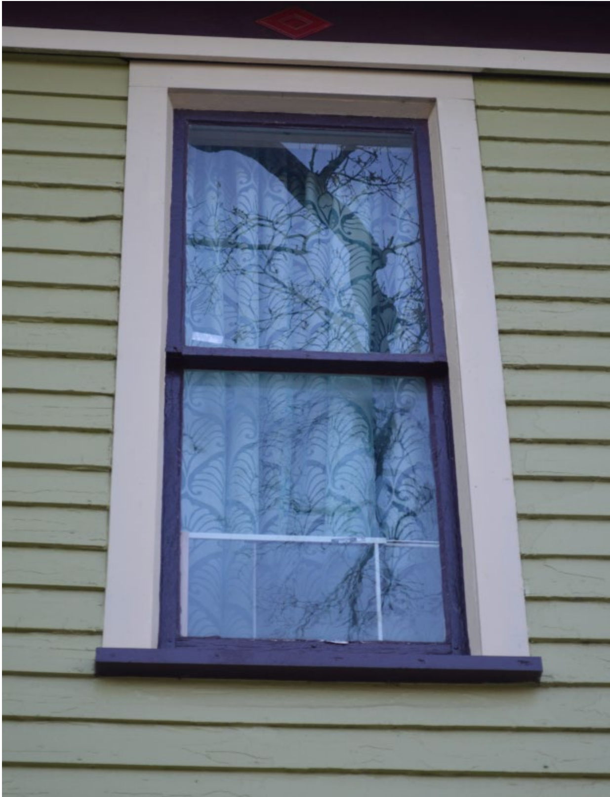
29"x70" double hung window among the four proposed to be replaced on second floor
