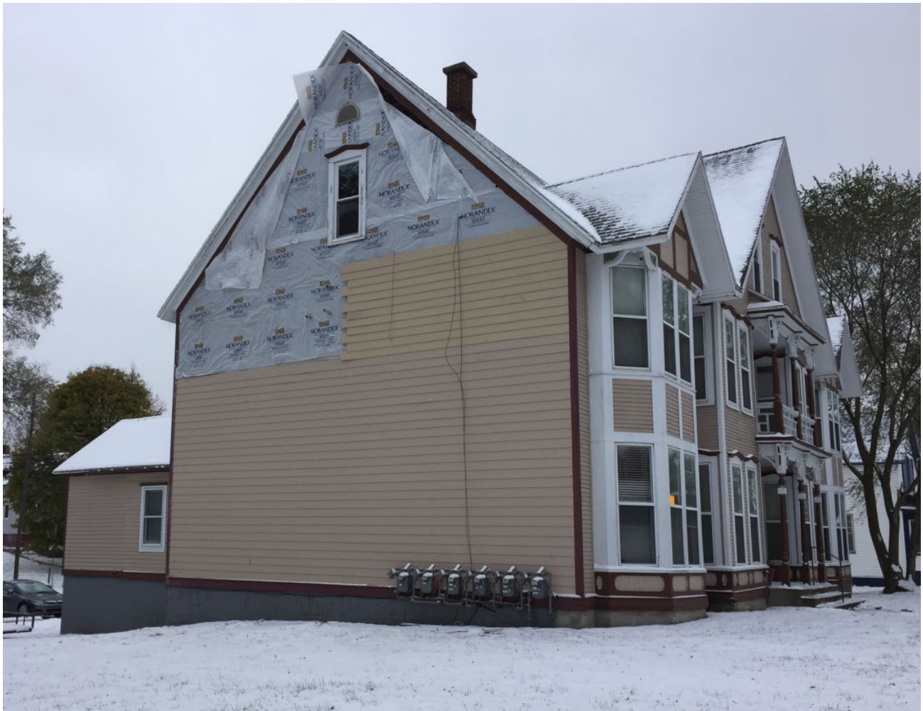
Northwest façade of 427 W. Muskegon Ave.
