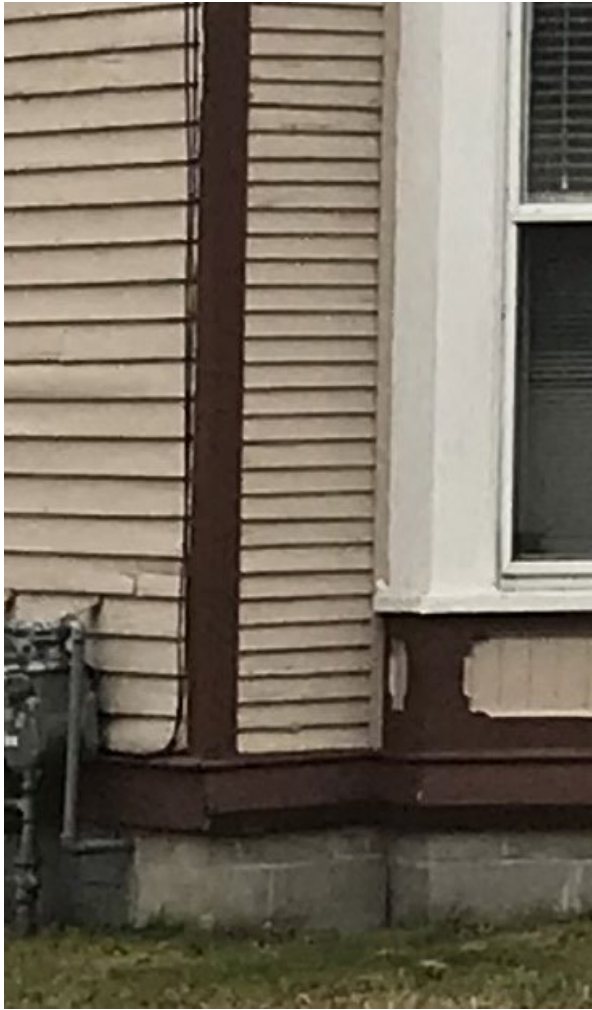
Northwest corner of structure before residing
