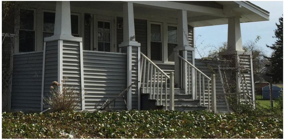
Appearance of front porch, prior to move
