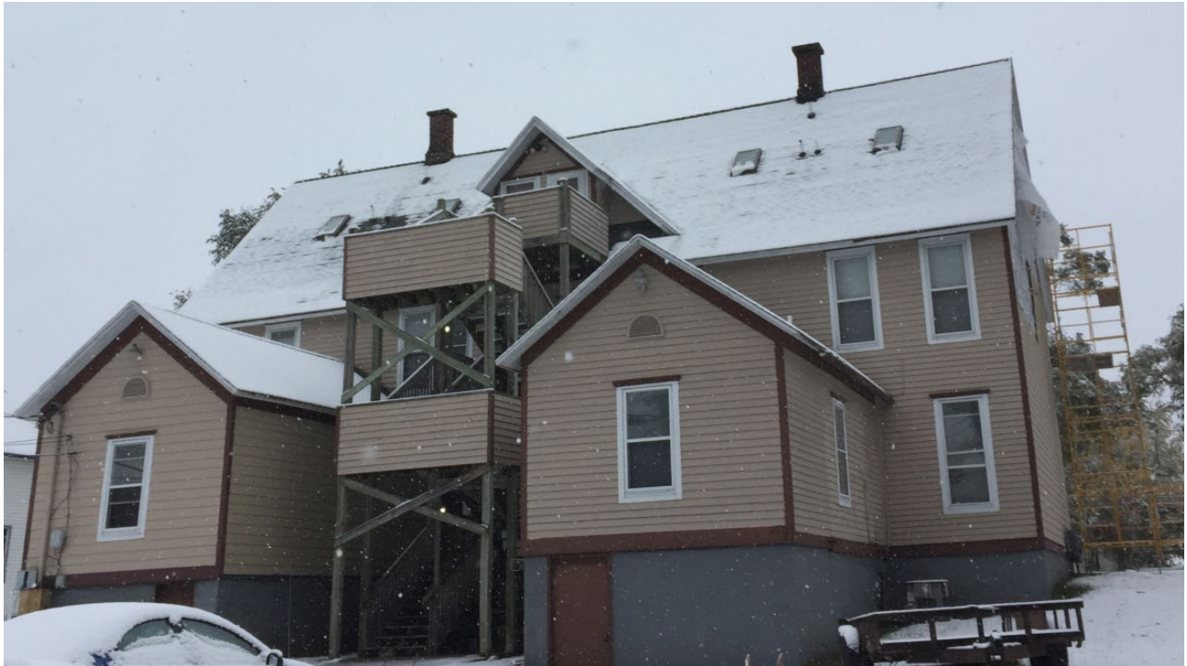
View of 427 W. Muskegon from alley (looking west) showing new siding on rear of structure
