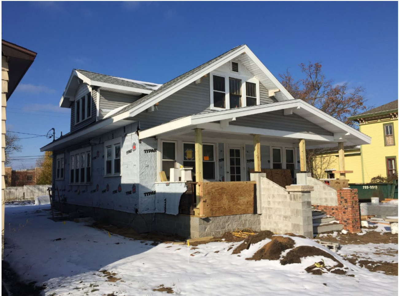
View of house from W. Webster Avenue, the front pair of windows on the left side of the house are proposed to be eliminated. The proposed brick work has started on the right side of the front stair.
