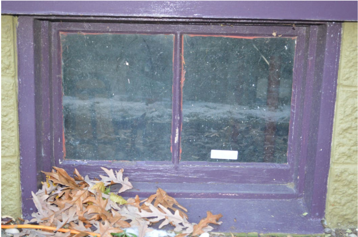
Basement window among the four proposed for replacement
