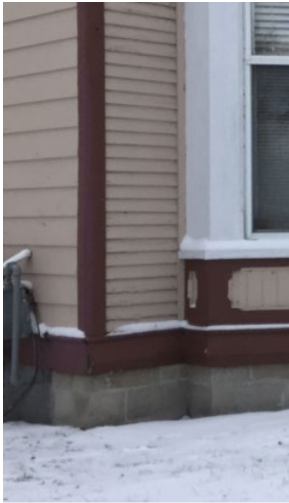
Northwest corner of structure with new siding visible at left
