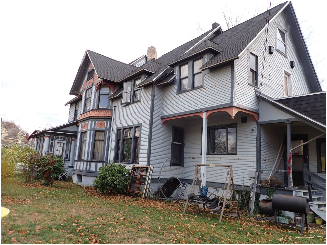
View of north (right) elevation from side yard.
