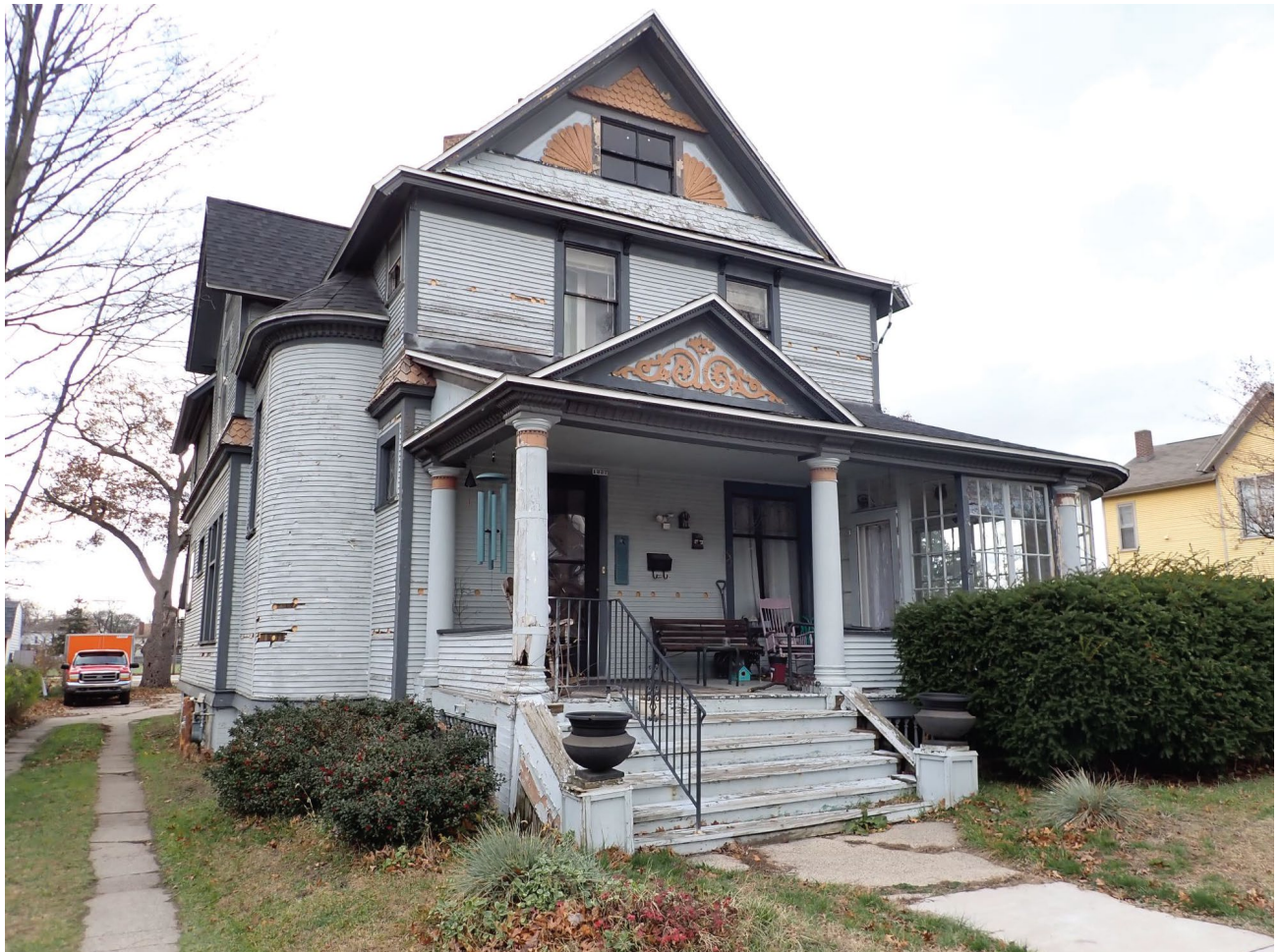
View of east (front) elevation from Peck Street.
