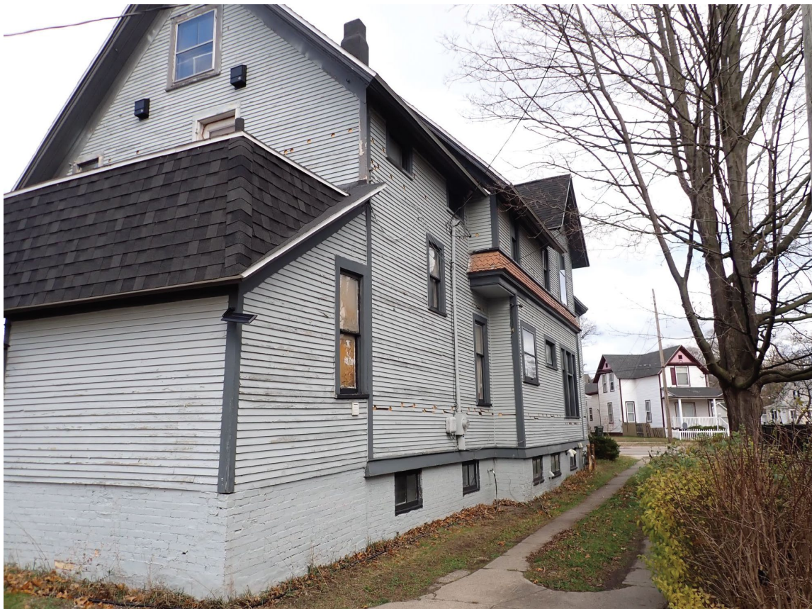
View of south (left) elevation from side yard.
