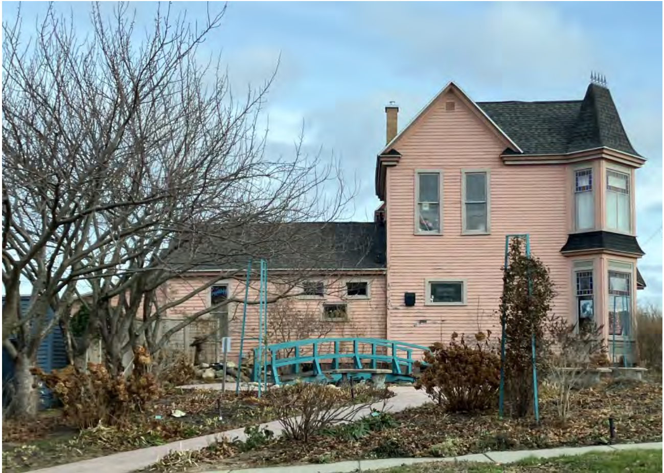
View of the side elevation from 5 th Street.
